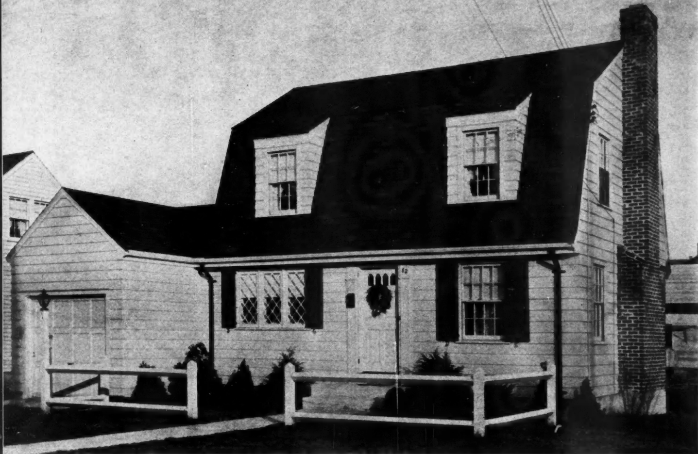
LOADED with Colonial charm, this little Dutch model was completed recently by Community Builders at West Hartford, Conn.
