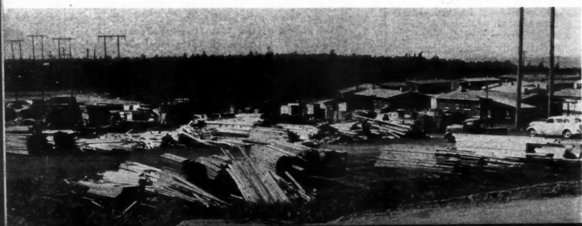
"CUT-UP-YARD" on Renton Highlands Housing Project where exterior wall sections, roof trusses, etc., are cut to measurement.
