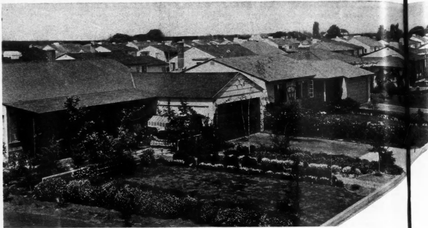
TOLUCA WOOD , one of Burns' recent Los Angeles developments where low-cost homes are set in charming landscaped surroundings. Thousands of similar homes have been built by private builders well within reach of war workers.
