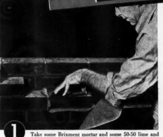
cement mortar. Try shoving a full head-joint with each mortar. You'll find that with the Brixment mortar (1), it is much easier to shove the brick accurately into place, with a full head-joint, than it is to do the same
