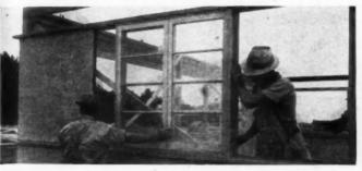
Wood casement window, complete with frame, is slipped into place. All elements are pre-fitted.
