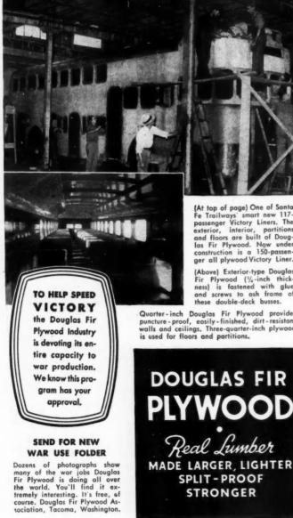
Fa Trailways' smart new 117-passenger Victory Liners. The exterior, interior, partitions and floors are built of Doug-las Fir Plywood. Now under construction is a 150-passenger all plywood Victory Liner. (Above) Exterior-type Douglas Fir Plywood (¼-inch thick-ness) is fastened with glue and screws to ash frame of these double-deck busses.
