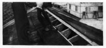
Celotex Celo-Roof combines insulation and roofing and is applied direct to roof trusses.
