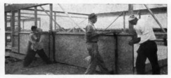
A sheet of  $1\frac{1}{2}$ " Cemesto is being applied to the lower section of wall. Panel is 12' long, 4' wide.
