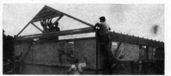
An end roof truss, equipped with ventilating louvres, is fitted into position in a matter of minutes.
