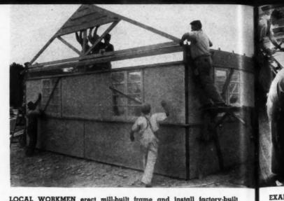
LOCAL WORKMEN erect mill-built frame and install factory-built panels of asbestos-cement and insulating board in war housing.
