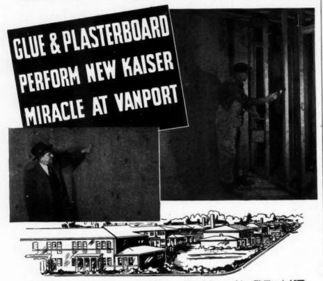
**RIGHT:** Brushing Laucks Construction Glue on studding before applying Wallboard. LEFT: Frank Stepanek, "expediter" of glue and plasterboard walls, for world's largest housing project.
