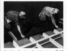
For New Roofs or Roof Repairs—Gold Bond Roof Plank is a heavy, durable gypsum board, which nails directly to wood joists and is quickly applied by any carpenter. Perfect base for builtup roofing.  $1\frac{1}{2}$ " and 2" thick, 24" wide and 8', 9' and 10' long.
