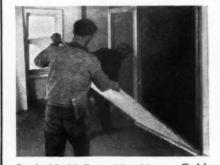
For inside Walls and Partitions—Gold Bond Solid Partition Panels are fastened between the studs by mouldings. Their large size means speed on the job. Their strength insures solid, rigid walls. Permanent or demountable and completely salvageable.
