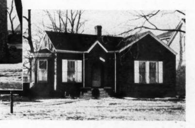
ABOVE and at right are shown the two sections of the house which was cut in two (see facing page). then both sections were rebuilt and brick veneered.
