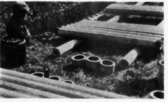
WOREMAN applying joint sealing compound to asbestos-cement conduit.
