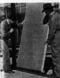
THE insulite surfaced panels are easily slipped into place; workmen here are starting at the corner with the first wall panel. (Note how bottom fits into grooved, built-up plate.) THIS peaceful Lexington, Mass., home designed by the well-known architect. Royal Barry Wills, is typical of expected post-war quality in planning and construction; comfort and stability will be sought.
