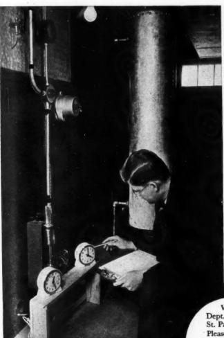
Checking time elapsed for various stages of fire during test period
