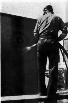
SHOT FROM A GUN—Workman above is demonstrating the new Colburn system of construction for low-cost fireproof housing. He is applying concrete to mesh over pan forms with new open hopper pneumatic gun developed by Construction Machinery Co.
