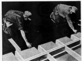
SYNTHETIC LUMBER-These men are putting on a new gypsum roof plank which, when nailed to wood joists, is an excellent base for built-up roofing. It was developed by the National Gypsum Co., to help relieve the lumber situation, has saved much precious time in getting many war plants into production.
