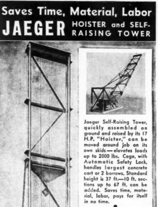
Labor scarce? This outfit can do work of 10 to 12 hodders with only 2 wheelers and a hoist operator. Speeds placement, too.
