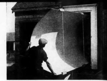
IN CONVENTIONAL CONSTRUCTION, use of "U" clan enables two men to quickly handle a full-wall size panel. Large sizes easily go through an ordinary door opening 2' 6" x 6' f" and through an open stair well.
