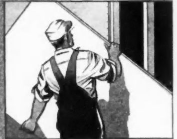
On outer walls, Insulite Bildrite Sheathing. The large boards provide a wind-proofed, water-proofed, weather-tight wall. Bildrite Sheathing has a bracing strength four times that of wood sheathing, horizontally applied.
