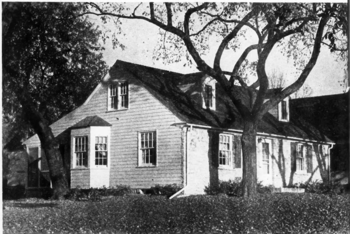
IMPROVED five-room design has added closed-in porch, stone veneer front and extra space on the second floor for two bedrooms and bath
