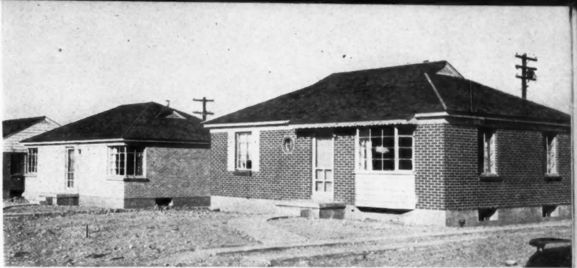
FHA TITLE VI war homes in Salt Lake City feature semi-modern designs with large bay windows, brick exteriors. Many have been successfully intermingled with Title II jobs in several good residential areas.
