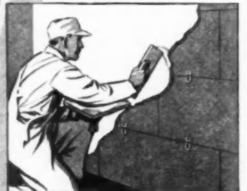
On inner walls—Insulite sealed Lok-Joint Lath, furnishes a second wall of insulation. The patented "Lok-Joint" provides a strong, rigid plastering surface, prevents joints from opening under trowel pressure.
