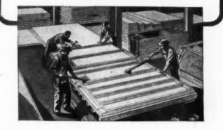
PREFABRICATION started with the question—"How can we build a house with sectionalized, factory-built, standardized panels?" *Precision-Built Construction* started just the other way around— "How can we build sectionalized panels to execute *any design?*"
