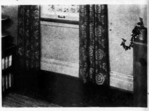
"Baseboard radiation" is the term commonly applied by the Crane designers to this new development, since the heat is introduced through continuous radiant panels that replace the conventional baseboard in the room. This new panel heating system has been under test for several years in actual installations.
