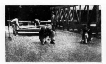
This essential plant is only one example among thousands where fireproof Gold Bond Gypsum Boards have licked the lumber shortage and helped the war effort. In this case it's roof plank, applied quickly—no waiting for materials to dry before applying the roofing material. Gold Bond Gypsum Exterior Boards do the same sort of job for outside walls . . . forming sheathing and finish in one operation!
