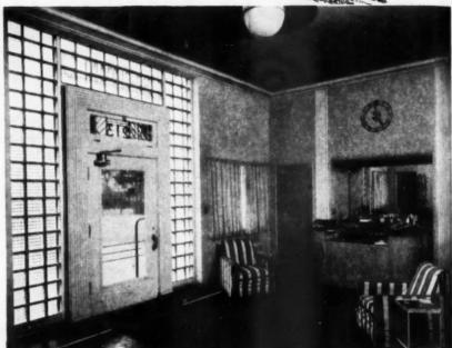
In Stores - Panels of Insulux can be used to flood salesrooms with softlydiffused natural daylight.
