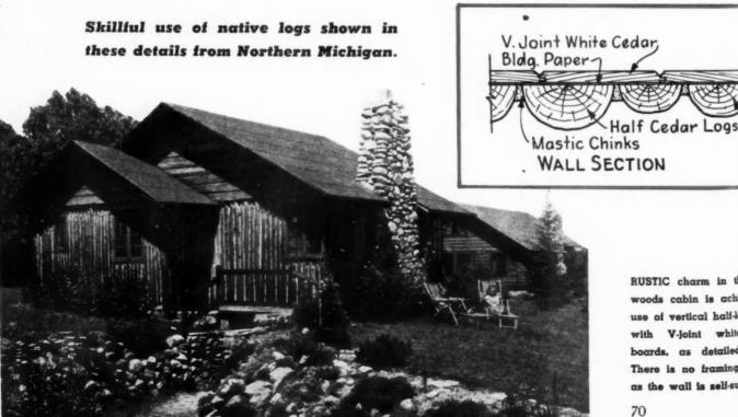
RUSTIC charm in this not woods cabin is achieved if use of vertical half-logs list with V-Joint white cold boards, as detailed chess There is no framing needs as the wall is self-supported
