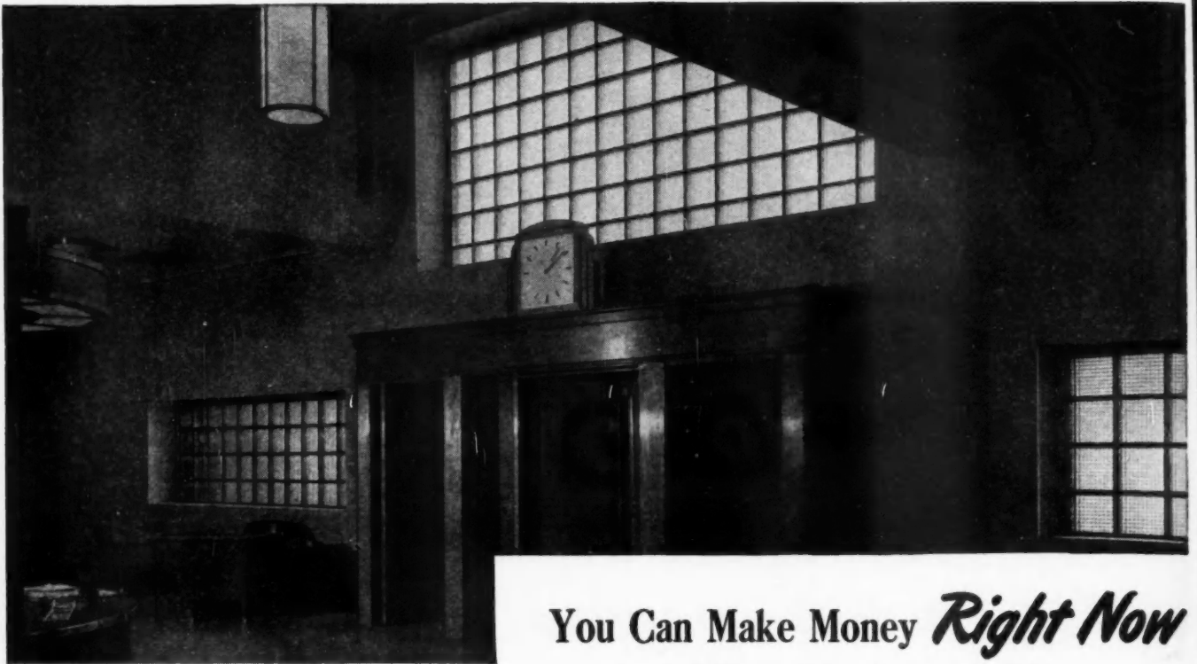
Building Managers use panels of Insulux to light up corridors and hallways and to transmit daylight from office to office.
