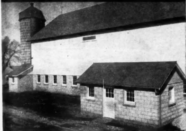
Old dairy barn with new concrete foundation before application of cement asbestos siding to walls. Concrete masonry milk house in foreground.
