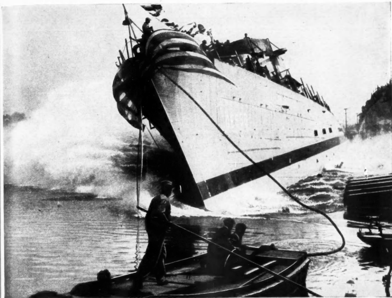
A Destroyer-Escort hitting the water from the Defoe launching ways
