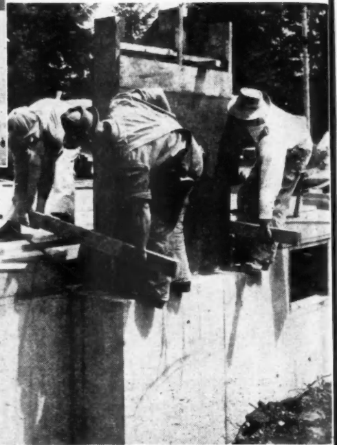
INGENIOUS plywood core is used for pouring the fireplace ash pit, at a saving of about $30. Photos show workmen lifting out the core form. Top view shows Contractor Miller pointing out to an "American Builder" editor the details of the ash pit recess in basement wall.
