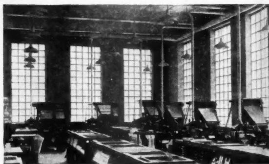
Manufacturers use panels of Insulux to solve troublesome problems of light, temperature, humidity and dust control.
