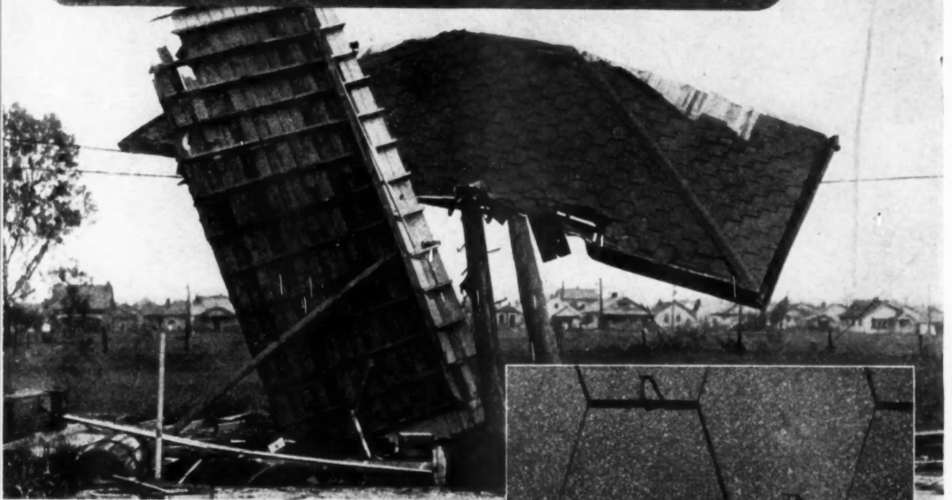
Photograph of roof deck blown completely off the house but with practically every Cyclone shingle intact.
