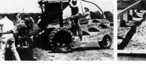
CONCRETE LOADED AT CENTRAL MIXER is carried in a Mixermobile buggy for pouring into foundation forms; 48 hours later forms are stripped, walls sprayed with a seal cure.
