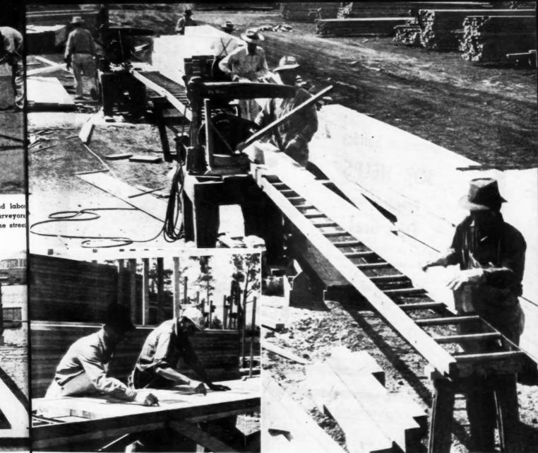
PRECUTTING AN IMPORTANT STEP as shown above. In insert, two workmen near stock pile are multiple marking studs for win-4 PRECUTTING AN IMPORTANT SILF as shown above. In insert, two workmen near store put one two cuts can be made without dow, door openings, partitions, etc. From there framing is passed along to the cutting line where two cuts can be made without as the store put of a cutor is an how with a store such as this.
