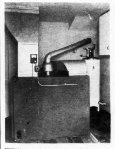
UTILITY room has efficient conditioner with supply trunk over ceiling joists; other equipment-heater, storage cabinets and washer.
