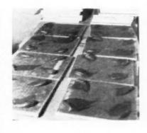
cement, such as the Armstrong installation specialists have devised for their own Cushiontone acoustical tile. The illustration shows how the four corners of each tile are daubed with cement before being applied to practically any flat, even surface. Such tiles weigh only between 8/10 to 1 3/10 pounds per square foot depending upon the thickness, which varies from 1/2 to 7/8 inches
