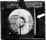
Wall-mounted fan, equipped with either fixed louvers or automatic metal shutter.
