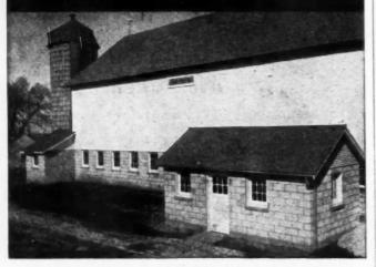
dairy bern with new concrete foundation before application of ostos siding to walls. Concrete masonry milk house in foreground. Better than new with concrete foundation and cement asbestes siding, this dairy barn is new a valuable farm asset.
