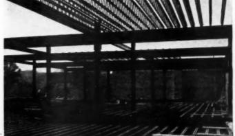
Ceco open web steel joists provide fire resistance and low maintenance cost.
