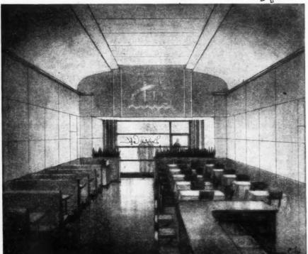
In the illustrated application above, notice that a curved treatment is used on the ceiling. Douglas fir plywood is ideal for such use, for it can be bent to simple curves without steaming and without danger of splitting.
