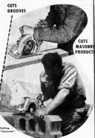
It's no news that SKILSAW is the finest timesaving tool you can own for making all the ordinary cuts in lumber. But there's lots of other work that SKILSAW can do . . . and do it faster, easier, better. Grooving, for instance . . . cutting sheet metals, compositions, asbestos cement and all masonry products . . . just an example of many unusual cutting jobs where SKILSAW can help you build faster and more profitably.
