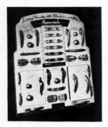
Two model operating doors which are a part of the demonstrator can be opened and closed to test the easy operation of catches and hinges. They also show how hardware is applied to both flush and offset doors.
