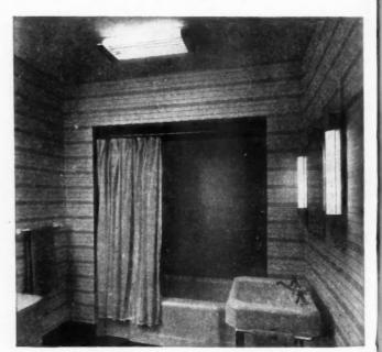
Note compact central fixture. Illustrates trend of designs in utility areas. Gives entire bathroom a soft, cool, shadowless light. Lamps on sides of mirror provide excellent illumination for shaving or applying makeup.
