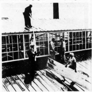
formerly used, had to be replaced at intervals of eight months. Before this aluminum roof was put on, test panels of aluminum were exposed to the cast house conditions for more than a year, showing no appreciable effects from corrosion.
