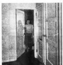
MODERN 3-panel door is cut to exact dimessions, machined and ready to hang before leaving factory.
