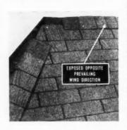
Plan courses so nails at ridge are covered by at least 1" of overlying ridge shingle. Last course of roof shingles may be turned over or trimmed even with ridge. Shingles at hips should be trimmed even with hip line. For cover shingles on ridges and hips, use Master-Bilts cut in thirds and trimmed to edges of "cutouts". Lay with butts exposed 5" to weather. Place nails 11/2" from each side, not over 6" from butts. On ridges always expose opposite prevailing wind direction.
