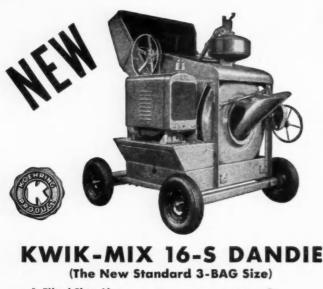
✓ Tilted Flow-Line Discharge Chute = Faster Discharge
