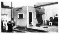
A Minnesota auto service man is proud of this small building. Walls constructed with Celo-Siding.
