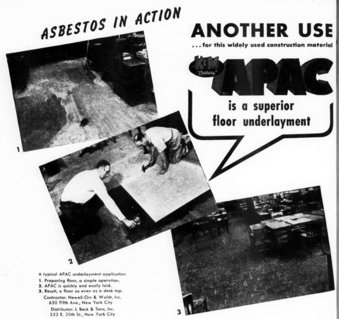
IN ADDITION to APAC'S many other uses, this versatile Asbestos-Cement Sheet Material has special features that make it ideal for flooring underlayment work. It provides a smooth plane surface for linoleum or resilient tile where subflooring is rough and uneven and must be leveled beforehand.
