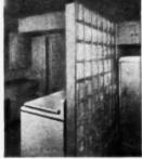
An Insulux partition is often installed in a kitchen to separate the cooking section from the refrigerating section.
