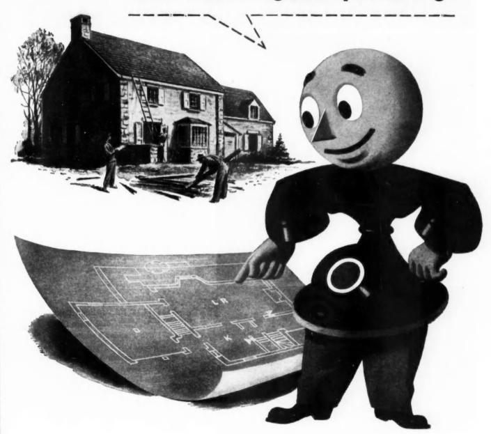
Even though some people are still waiting for telephones, alert architects and builders are not forgetting to plan for the days when they'll be available without stint. Built-in telephone facilities—with conduit concealed out of sight in the walls and neat outlets all ready for connection—add much to a house at little cost.
