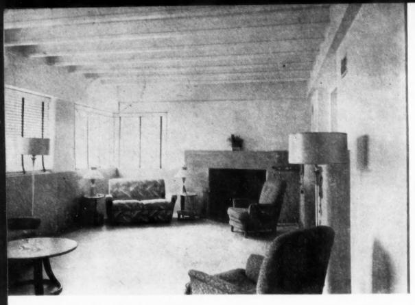
LIVING ROOM of Hasdonfield, N.J., home show, ing exposed Lith-1-Bar joist ceiling, eliminating the cost of ceilings and providing an excellent acoustical effect. All first floor level floors have I inch of terrazzo finish as poured on Lith-1-Bar joist, providing an attractive, permanent type of floor.
