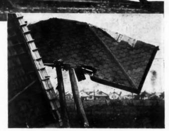
Roof deck blown completely off, but with practically every Cyclone shingle intact.
