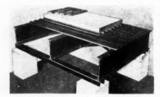
Joists are screwed to channel plates. Clip-on bridging supports the joists. Steel sheathing, over which concrete is poured, is nailed to the joists and hardwood flooring then is laid on the concrete.
