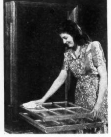
The weights, chains and pulleys have been replaced with a new patented device which provides smooth, noiseless and non-rattling up and down movement.
