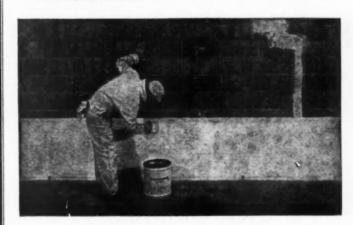
a. THOROSEAL, a slow-set hydraulic compound, gives the applier 8 bit & nows, before set begins, to brush THOROSEAL into the masoury surface. (Serubhing not necessary, as THOROSEAL is prepared especially to now easily and quickly into every crack, void and defect in the surface, where it becomes structurally stronger than the surface to which applied.
