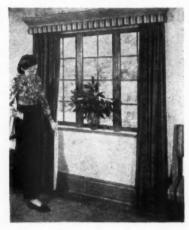
Replacing the conventional wooden baseboard, the new heat panel delivers radiant heat rays into the room at ankle height. In appearance it is a hollow cast iron unit 7 in. high and 13/4 in. wide, connected with the usual heating boiler. The panels are installed on the outside walls in place of the regular baseboard and painted to match the woodwork of the room.
