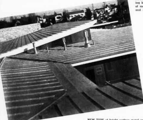
with Celotex insulation is used both parallel and perpen. Honeywell thermostats control even dicular to roof pitch. New type suction vents terminate below high point, temperature at all times. A Westing
