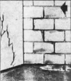
PROBLEM B: Water trickling through mortar joints, wall and floorline cracks, during and after rains.
