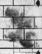
PROBLEM A: Dampness seeping through porous masonry surfaces like stone, concrete, coment or cinder block.
