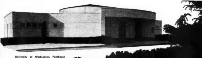
University of Washington Penthouse Theater, Seattle — a striking, attractive, all - plywood structure. Outside walls are of 3/8" Exterior type plywood over 3/8" plywood sheathing.
