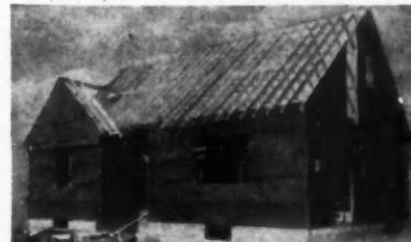
**CUTS SHEATHING COSTS 1/3 to 1/2.** One man can handle the 1/2"x2'x8' panels, cutting and nailing right on the studs. You can use brick, wood, asbestos, stucco or stone exteriors.
