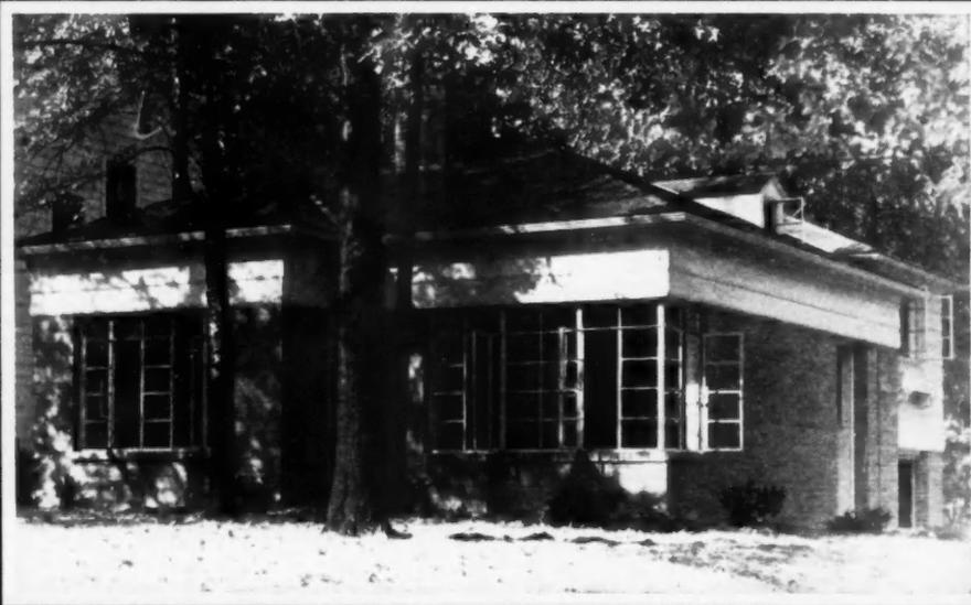
CORNER WINDOWS are featured in a large proportion of current plans, especially for small homes when the extra benefit of more unbroken interior wall space is particularly desirable.
