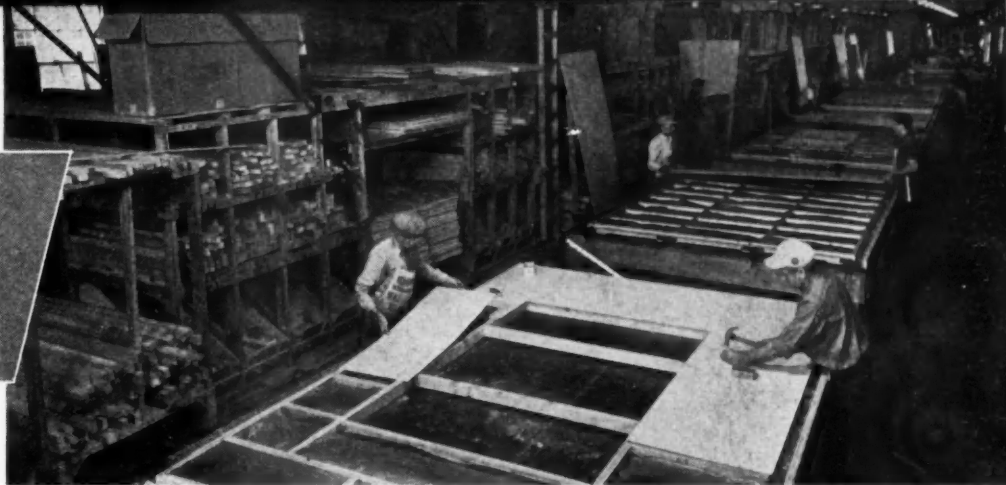
PRECISION-BUILT HOMES CORP. uses assembly line technique in fabricating wall panels.
