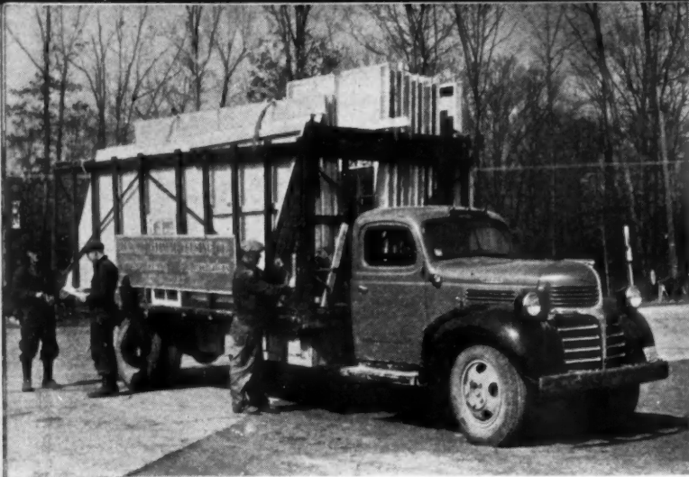
ECONOMY PORTABLE HOUSING CO. unit loaded on truck.
