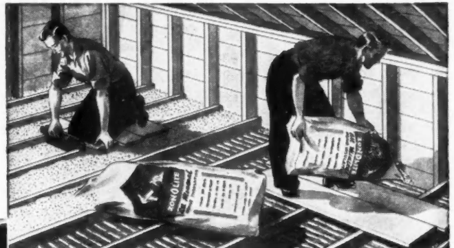
• Zonolite Granular Fill easily installed in attics and sidewalls—new work or remodeling. No gloves or masks needed.
