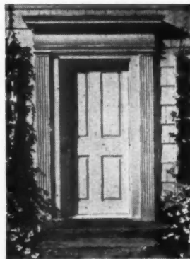
Curtis Entrance C-1730 recalls many fine doorways found in Connecticut and Massachusetts. Note the entablature with its bowed face, dentil course and pilaster beading. H. Roy Kelley, Architect.
