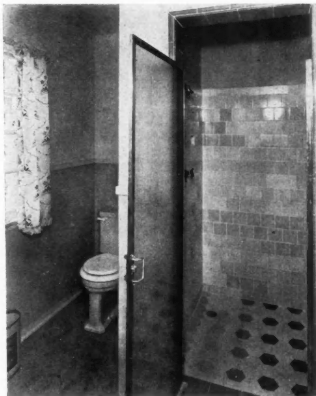
FEATURE of bathrooms is shower stall with tile walls, glass doors.
