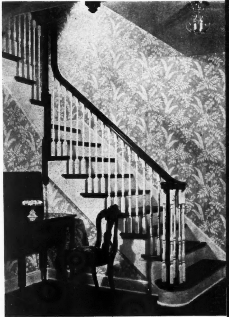
STAIRWAY has delicate balusters, mahogany finished handrail.
