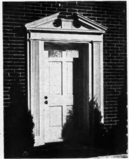
GEORGIAN entrance with broken pediment. Frame designed by H. Roy Kelley, architect.
