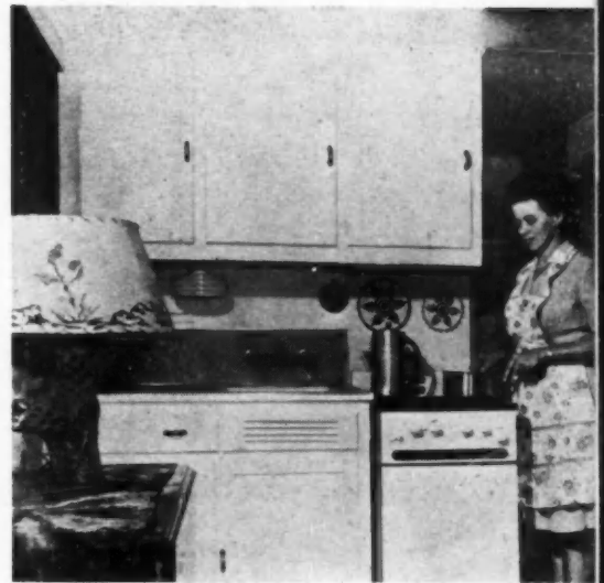
KITCHEN of Wingfoot Home is complete.
