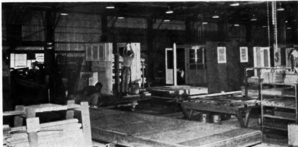
WINGFOOT HOMES (Goodyear subsidiary) uses dolly trucks to keep production moving.
