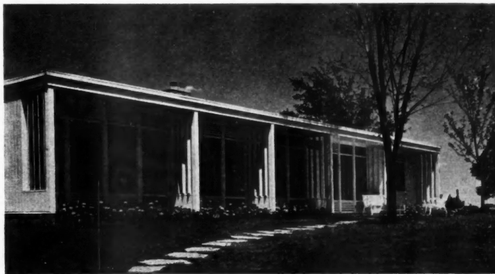
GREEN'S READY-BUILT HOMES has gained national attention with its Solar Home.
