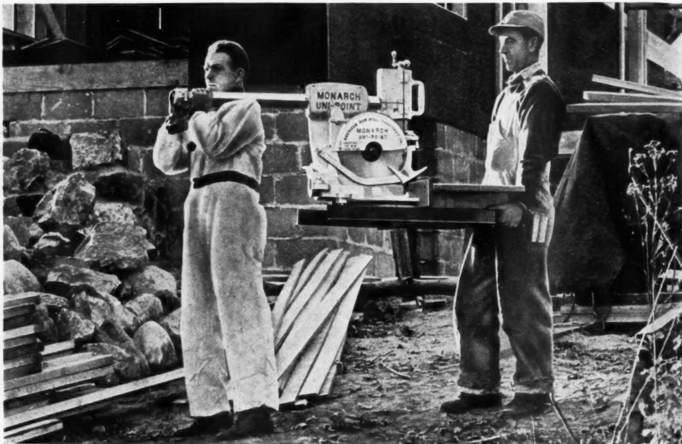
RADIAL saw weighs only 200 pounds and can be carried by two men.
