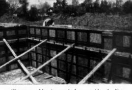
Alignment and bracing required on one side only, Note simplified method of inside corner and filler forming. Erected Panels are "clean"—offer very little obstruction.
