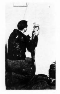
dust thus created in its own vacuum cleaner, a workman with this tool can install the necessary copper tubing inside a wall so that with the use of a plastic and masking tape the finished
