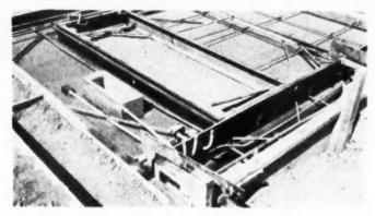
DETAILS of a 6 in. load bearing partition wall ready to pour. Outer or edge molds and door forms are of  $\theta$  in. steel channel iron.
