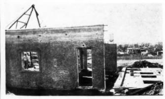
WALLS being lifted. Cast on the ground, they are in their proper place on being tilted up. Welded steel rods fasten the corners.
