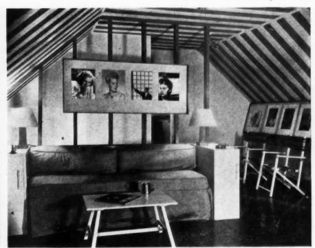
IN remodeling attic, open studwork was painted, chimney enclosed with insulating board.
