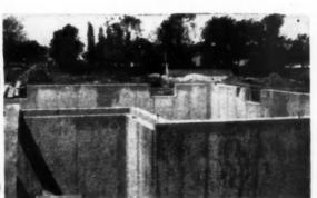
Smooth-surfaced, straight walls of uniform thickness—accurate inside and outside corners are assured on every UNI-FORM foundation. Boxing out and brick ledges are very easily handled.
