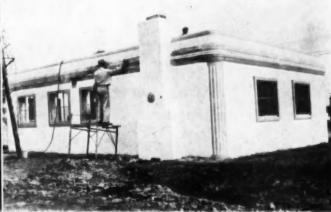
ABOVE: Front (left) and rear (right) views of the "plastic rock" concrete house assembled (erected) and ready for finishing work.
