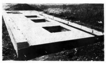
COMPLETE wall unit, including fireplace, ready to erect (tilt up). The foundation and the two walls are separated by air space.
