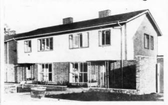
ONE of Britain's new steel and concrete houses, designed by the British Iron and Steel Federation, is shown above.
