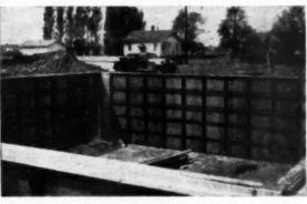
Concrete has been poured and Panels are ready to strip. Quick removal of cut nails from Tie ends releases Panels.
