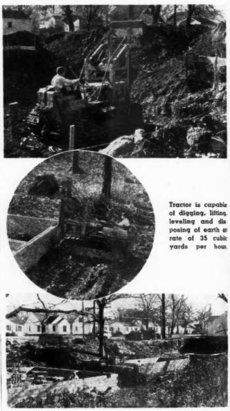
THIS small model track-type tractor can excavate two basements a day.
