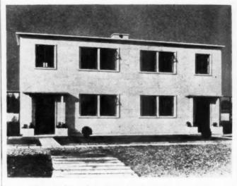
ABOVE: "The Orlit House" uses precast concrete beams to form a reinforced concrete monolithic frame.
