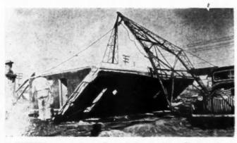
A TWENTY ton exterior wall is tilted into place. The triped derrick, operated by a winch truck, lifts the wall in four minutes.
