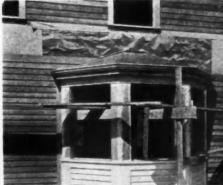
Copper armored Sisalkraft flashing applied at roof and sidewall juncture.
