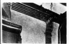
Typical installation of copper pipe and fittings with soldered connections. Photo: Mueller.
