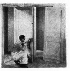
Pre-fit doors eliminate cutting, fitting.
