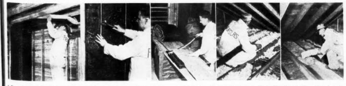
aft to right: Ceiling job with batts; roll blanket going in sidewall; recommethod of cutting roll blanket; ceiling application of blowing
