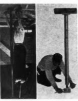
Adjustable steel columns correct sagging floors. Photo: Perma-Jack.
