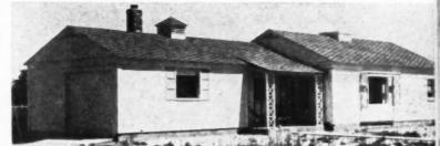
Flat asbestos-cement board covers sidewalls. Photo: The Ruberoid Co.
