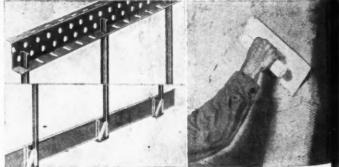
Metal ceiling runner, studs, and base clips for 2-Inch solid plaster partition. Photo: National Gypsum.
