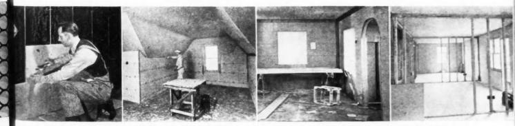
Left to right: Application of Nu-Wood insulating board lath; plastering over Insulite's plaster base with metal clips between studs;
