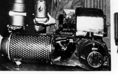
light-weight simplified conversion oil burner compared New with 1925 model having 480 parts, weighing 320 pounds. Photo: Timken Silent Automatic Division, Timken-Detroit Axle Co.
