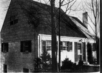
Recently developed and improved products shown here include asbestos shingles, asbestos siding shingles and waterproofed concrete block sidewall. Photo: Johns-Manville.
