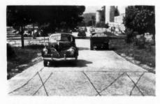
Scaling indicated on normal slab in foreground. Air entraining on balance was scale resistant.
