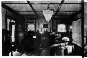
Example of fiberboard installation of the early '20's. Note how moldings contrast sharply with panels. Photo: Upson Co.
