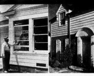
Drop siding with metal corner joint covers provides permanence.
