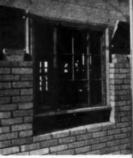
Brick veneer over wood sheathing with a metal casement.
