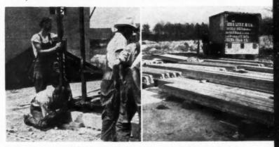
Welder anchors steel frame assembly, Precast concrete joists ready for to joists. Photo: Great Lakes Steel Corp. delivery. Photo: W. E. Dunn.
