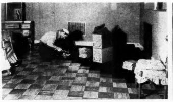
Method of applying prefinished block flooring to wood subfloor is indicated in this illustration. Photo: E. L. Bruce
