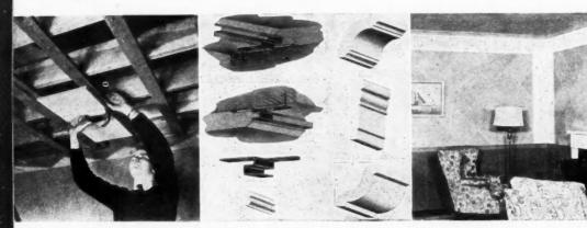
Left to right: Applying insulating board tile with concealed metal clips; detail of metal clips and decorative wood molding; finished job with insulating board tile on ceiling and sidewall; sidewall finished with insulating board plank. Photos: Wood Conversion Co.
