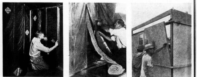
Wood fiber blanket insulation showing typical installation. Photo: Wood Conversion Co.
