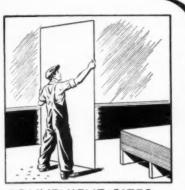
CONVENIENT SIZES Supplied in handy 4' x 8' sheets, in thicknesses of <sup>3</sup>/<sub>1</sub>e<sup>4</sup>, <sup>1</sup>/<sub>4</sub>", <sup>3</sup>/<sub>8</sub>".
