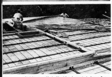
Steel beams combined with reinforced concrete to form a floor. Finished floor will be wood block or lineleum. Photo: Jones & Laughlin.
