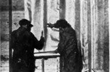
Flaked aluminum bonded to Sisalkraft to form reflective insulation and vapor barrier.
