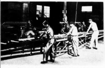
Precutting on production line with series of Walker-Turner radial power saws.
