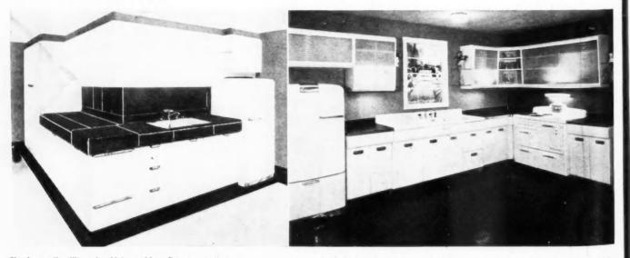
The Ingersoll utility unit which combines fixtures, appliances, and fittings of kitchen, bathroom, laundry, heating, plumbing and electrical lines in a compact central steel core.
