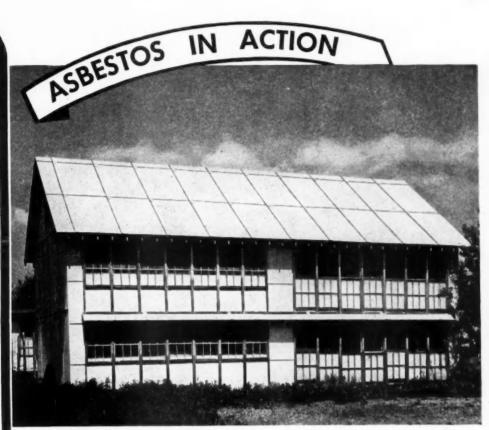
This modern two story poultry house - of unit design - has a roof and sidewalls of Apac, making it resistant to fire, pecking, weather, termites, rodents.
