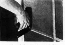
Installing plastic screen with small stapling machine. Photo: Monsanto Chemical Co.
