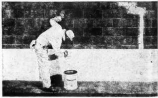
B. THOROSEAL, a slow-set hydraulic compound, gives the applier 3 to 4 hours. refore set begins, to brush THOROSEAL into the masonry surface. (Scrubbing not necessary, as THOROSEAL is prepared especially to flow easily and quickly not every crack, void and defect in the surface, where it becomes structurally tronger than the surface to which applied.)
