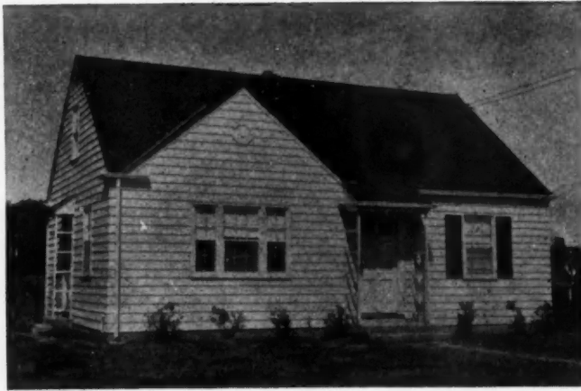
ABOVE: One of the Pomeroy-American Houses completed homes.
