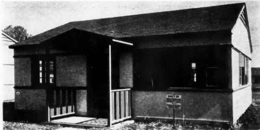
BULK of the houses will be these five- and six-room Cemestos.
