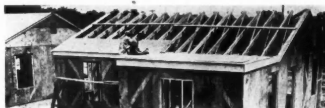
FOURTEEN Teco truss rafters eliminate bearing walls.
