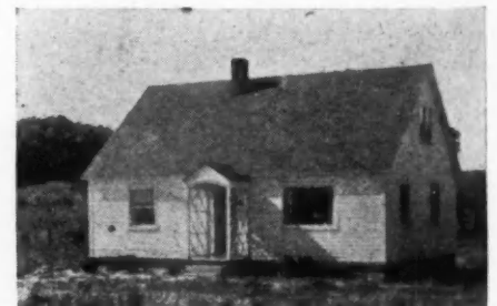
NEW Johnson home is simple, compact. There are two extra bedrooms on second floor. Roof is of thick-butt, asphalt shingles; asphalt felt over sheathing acts as insulation.
