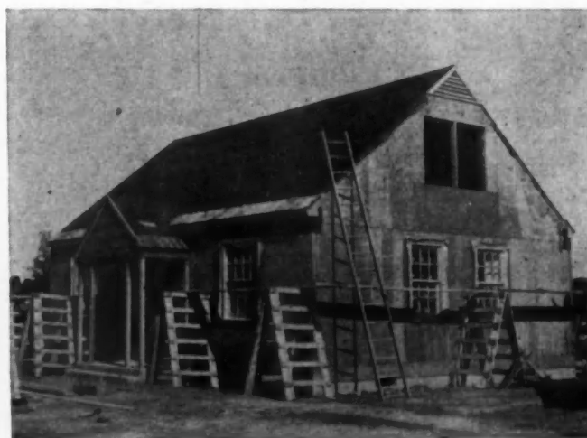
WOODRUFF firm uses "convenience horses" in place of scaffolding.
