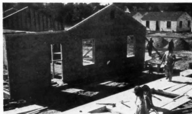
GOOD supply of portable power hand saws speeds work on site.
