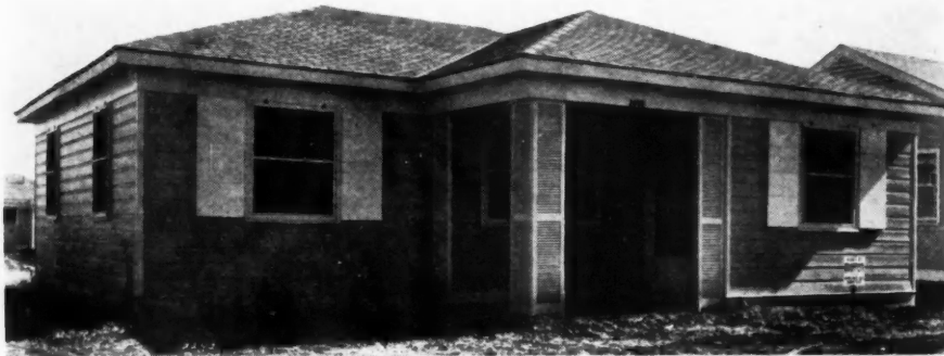
ONE of the twenty-two Crawford prefabricated houses which have been erected.
