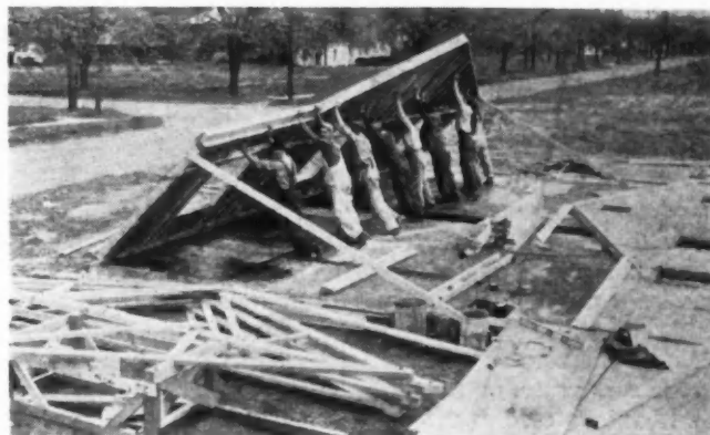
GABLE end wall being raised. Opposite end ready to raise.
