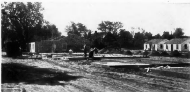
CREWS assembling and erecting exterior walls on slabs.
