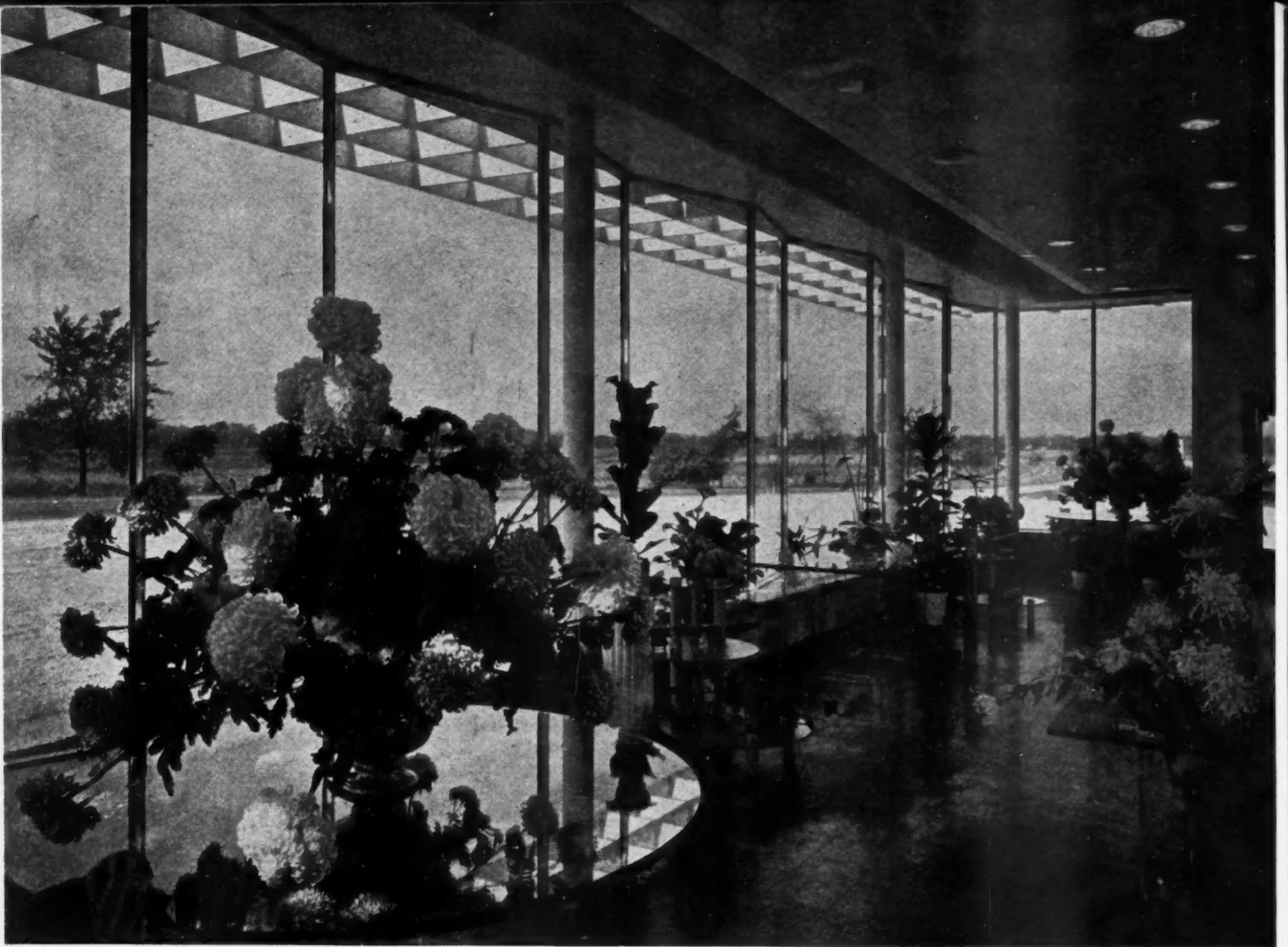
THE absence of extended bulkheads under window wall permits great flexibility for interior arrangements. Photos by Hedrich-Blessing Studio.
