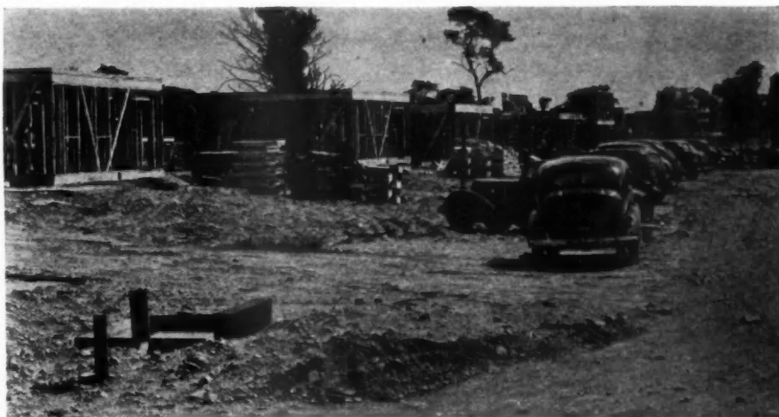
CONSTRUCTION scene above clearly shows assembly-line technique used in framing.
