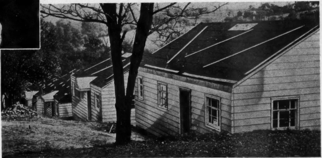
GENERAL view of partially completed units after application of aluminum siding.
