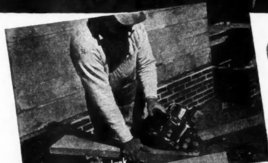
45° Angle cut—2" plank
