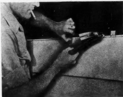
SIDING is nailed to building with clips.
