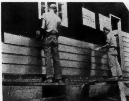
WORKMEN lock each piece to the one below.
