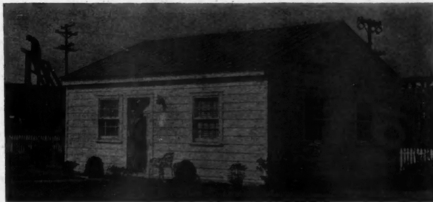
COMPLETED Southern States' all-aluminum house with clapboard style exterior wall sheets.
