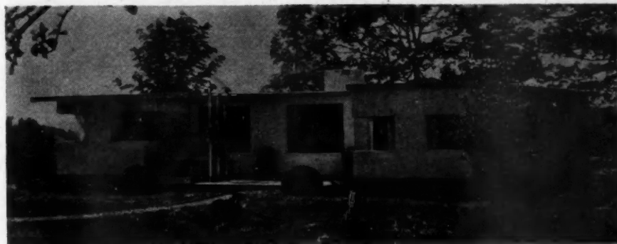
ALUMINUM coated plastic panels two inches thick, 4x8 feet, form walls of this house.
