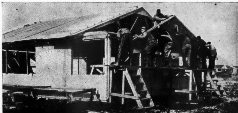
INSULATION being applied to wall sections, under roof, using assembly line methods. Below is shown a pre-assembled section being erected by workman after delivery to building.
