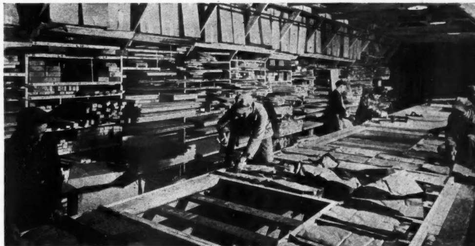
INSULATION being applied to wall sections, under roof, using assembly line methods. Below is shown a pre-assembled section being erected by workman after delivery to building.
