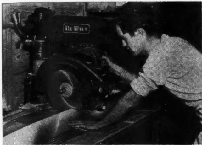
Radial saws equipped with special blades cut the new aluminum siding easily and accurately on the job, speeding work with this new material. Photo: DeWalt.
