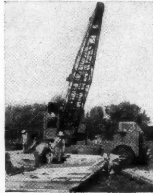
Power equipment is on the job in prefabrication. Photo: Harnischfeger.
