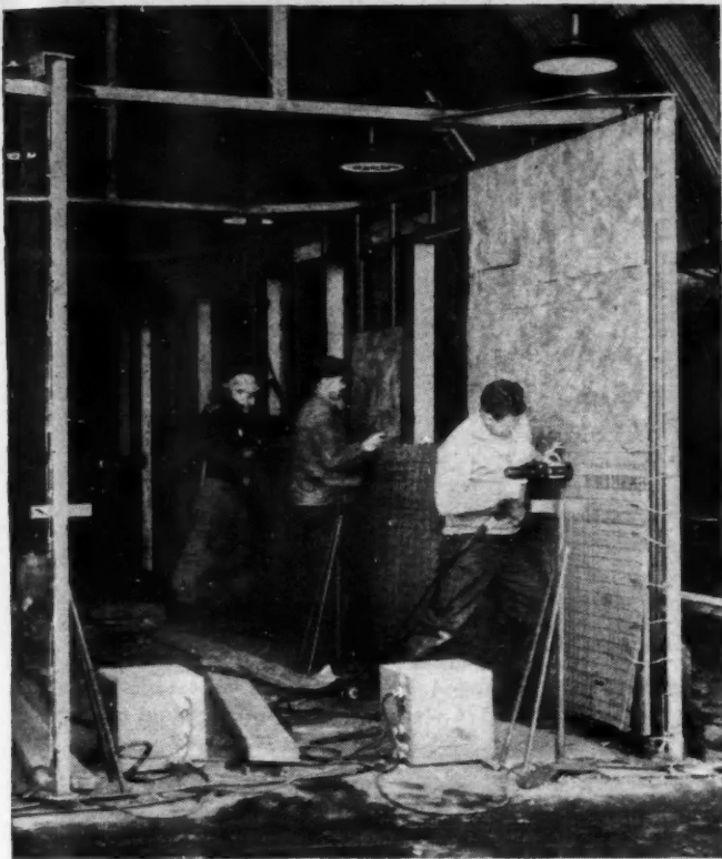
STUD-WELDING insulation and metal lath to exterior of steel frame.
