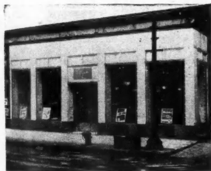
THE old building before work was started on the $125,000 remodeling project.
