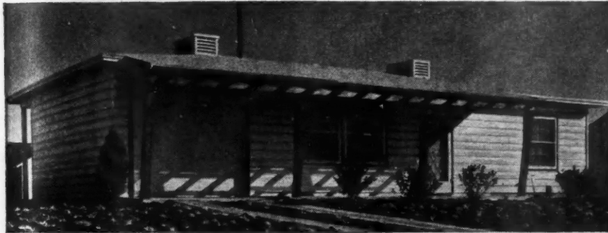
FRAMING on Southern Builder homes is nailed up with ring shank nails. All parts prefit.
