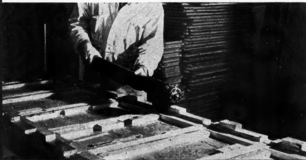
IN assembly of built-up plywood wall sections the glue gun plays a prominent part. Below is automatic nailing machine securing plywood to wood frame until glue has set.
