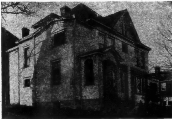
The above photograph shows the same stucco home after it received one heavy application of THOROSEAL, which, after being applied for one year, shows no leakage or dampness on the interior of the building.
