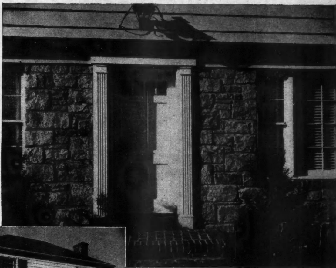
DETAIL of the front entrance and the adjoining stonework of the house shown below. A well proportioned and effective overhang of the second floor is a feature of the front wall of house.
