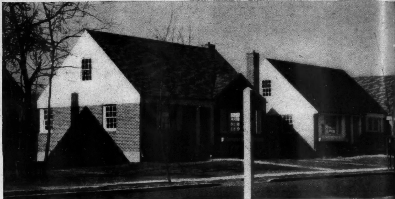
THE houses shown in the street view above, each with a different exterior treatment, spring from one basic floor plan.
