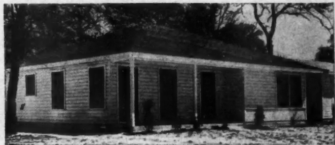
PLUMB & Mitchell are finishing up 250 in Southern Village.
