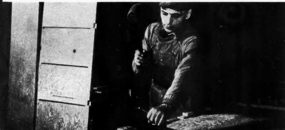
IN assembly of built-up plywood wall sections the glue gun plays a prominent part. Below is automatic nailing machine securing plywood to wood frame until glue has set.
