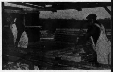
WALL and root sections are site fabricated, ready for assembly.
