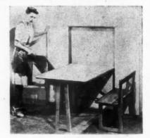
In new construction, the Foldinette can be recessed into a standard 4 in. wall by framing around the cabinet and fastening to studs and header.
