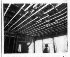
HEATING coils installed in ceiling ready for installation of metal lath and plaster.
