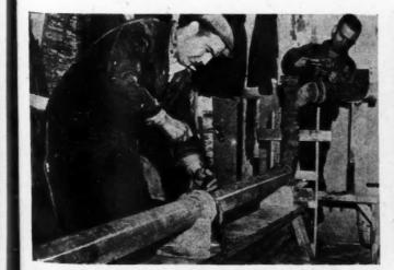
PLUMBING and heating assemblies are shop fabricated and tested.
