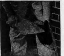
ld be thrown on the end Plenty of mortar show of the brick to be place
