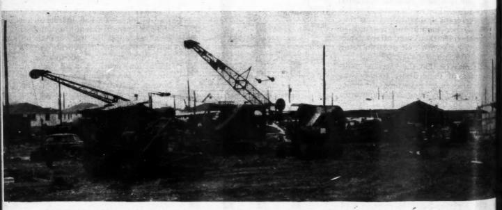
DRAGLINES, buildozers, ditchers, back-fills and portable generators owned by Kelly-Generes, used for site preparation.
