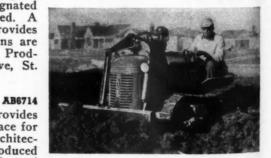
to operate close to the walls of houses and make close turns around trees, thereby accomplishing work which formerly required hand labor. The dozer is hydraulically operated with raise, lower, floating and hold positions, and is easily transported.
