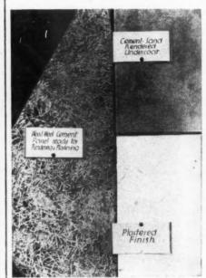
MADE of a cement, sand and wood fiber mixture, this wood-wool plate panel is sultable for exteriors and interior linings.
