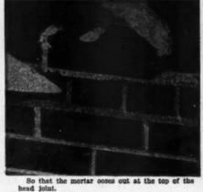
All head joints in both face brick and back-up work should be completely filled with mortar. One good method for doing this is to throw plenty of mortar on the end of the brick to be placed. (This should be done in such a way that the mortar is scraped off the trowel by the bottom edge of the end of the brick.) Then push the brick into place so that the mortar oozes out at the top of the head joint.
