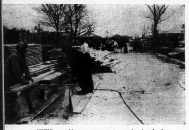
USING portable power saws to cut framing lumber.
