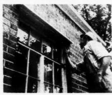
AB28105—The Aluminum Building Products Co., East McKeesport, Pa., announce the "Lewshield" window and door cap, rigidly made of aluminum alloy in a neat and pleasing ornamental design. The item is made in two widths—4 inches for small openings and 5½ inches for larger openings. Both are available in standard sizes or may be obtained in any special length up to and including 21 feet, adaptable for all different styles and types of windows.
