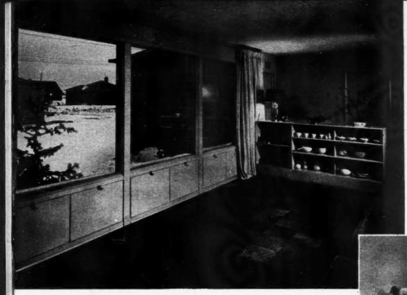
HASCO block flooring in place in living room. Blocks were laid directly on concrete with mastic. Note pleasing pattern resulting from red oak grain in blocks. Below, laying flooring on coment slab with mastic
