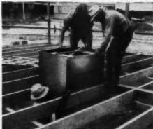
Easy, economical installation. This photo shows a Coleman Floor Furnace in place—in the floor, not on it and not in the basement. No basement is needed, so often you can save the cost of excavation; and you save much costly duct work. Easy to connect with chimney and fuel line. Models from 25,000 to 70,000 BTU input or equivalent; single or multiple installations.
