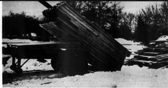
TRUCKMAN chains free end of load at site, and drives off. Load is dropped as a unit. Square end of load lets thin boards hit together
