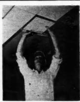
AB28155 — A light-weight, low-cost acoustical tile with high sound-absorbing properties for ceilings is announced by Owens-Corning Fiberglas Corp. Painted white at the factory, the tile has a felted fiber surface and is beveled on all four edges. It can be cemented to a solid backing, or it can be mechanically mounted on wood.
