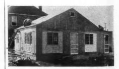
ROOFERS putting finishing touches on factory-built house held intact with glue
