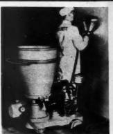
A82846—Colorcreting is a process of pneumatically applying a cementatious material to exterior and interior masonry surfaces. Colorcreting outfit consists of a mixing drill, compressor, electric or gasoline motor, a length of hose and a gun. Outfit and materials are available from Colorcrete Industries, Holland, Mich.
