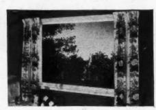
The popularity of the picture window is growing rapidly for both new work and remodeling. There are many possible combinations with Silentite windows flanking the stationary sash, or these sash are often used alone, as pictured above. This is Curtis Design C-2735 and is made in two sizes -5-0x4-6 and 6-0x4-6. This sash is shown on far left with double-hung Silentites on either side.
