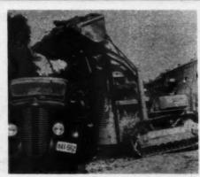
AB2811—The Caterpillar Tractor Company's diesel D4 track-type tractor, equipped with Traccavator, is utilized by builders to excavate foundations for houses and other structures at the start of construction work. When construction is actually under way, the unit is suited to numerous jobs on the site, especially for back-filling and leveling ground. This tractor is one of a number of units which are manufactured by Caterpillar Co, for use by builders.
