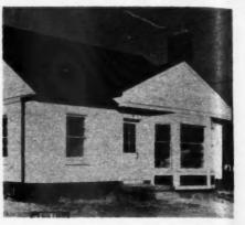
AB2875—Kimberly-Clark Corp., Neenah, Wis., has developed a plastic surfacing for plywood used in concrete forms. The surfacing multiplies the usefulness of the forms many times, in addition to making them easier to strip, faster to clean and holding the need for oiling for reuse to a minimum. This new plywood form material, which was used to build homes, like the one shown above, produces a surface smoothness equal to steel forms.
