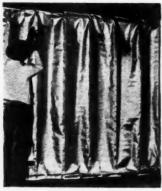
AB28167—A new method of obtaining dry walls in home construction is announced by The Sisalkraft Co., Chicago, III. It involves the use of Sisalkraft building paper over sheathing on the outside and the new Sisalation reflective insulation on the inside wall. Combination of the two minimize harmful effects from condensation.
