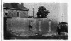
STARTED from framework in early morning, interior sections of this house are in place by 9:45 a.m., framework completed, and job taken over by roofers at 4:20 p. m.
