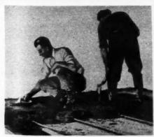
A828209—Zonolite Stabilized Concrete Aggregate is becoming increasingly popular to produce insulating concrete floors. When placed beneath radiant heat ducts or coils, Zonolite concrete prevents wasteful heat loss into the ground and facilitates wasteful heat loss into the ground and facilitates efficient and economical operation of the heating system. These floors have been widely used in rural, commercial, industrial and residential building, with or without radiant heating systems.
