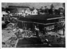
THE new material is poured in plywood molds which here have been placed, ready for the "Thermo-Con," After the material is poured in the forms it expands 125 per cent in 29 minutes, and attains rigid hardness
