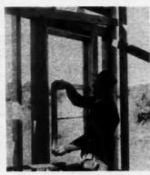
AB28183—Especially designed weather-strip to permit possible shrinking or swelling of the sash is a special fea-ture of Bilt-Well Superior unit wood windows made by Carr, Adams & Collier. In addition to easy operation the year round, sash may be re-moved without loosening or removing the weatherstrip. Easy to assemble.
