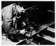
AB28126—Here is a tool designed for quick application of flooring, siding and sheathing with the tightest possible joints. Patterned on a lever principle, similar to a jack, it can force even bedly warped boards into line and hold them in position for nailing. A tap of the hammer against anchor sets tool into position on joists, and lever action squeezes the boards together. The fool is made by Maco Corp., Huntington, Ind.
