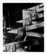
AB2803—The Trip-L-Grip framing anchor, made by Timber Engineering Co., develops double strength over customary toe-nailing of rafter-to-plate joints. Applied to the plate before installation of rafters and trusses, they automatically space roof members at required distances. The framing anchor may be used at all critical joint points.
