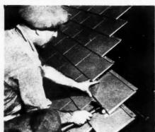
AB2813—Rustproof, fireproof, rotproof, Reynolds Lifetime Aluminum shingles eliminate maintenance. Their surface is raised away from the sheathing of the roof, providing an air space faced by aluminum, which reflects as high as 95 per cent of radiant heat from either direction. Easy to apply, because they are self-aligning, they can be painted or left unpainted, in which case, natural weathering tones down brightness.
