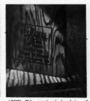
AB2871—This unretouched photo of Douglas fir plywood panels show clearly two of the industry grade trademarks for ready identification of types and grades of fir plywood. Upright is Plypanel Sound I Side grade interior type for use where one side is to be exposed. Horizontal is same grade exterior for use on outside sidewalls.
