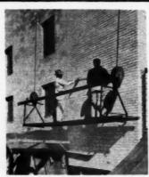
AB2811—Safway Steel Products, Inc. of Milwaukee makes this light duty swing stage, called Saf-T-Swing. It is designed especially for such jobs as maintenance work, painting, cleaning, tuck-pointing, etc. The new winch design increases safety. Two winches, entirely gear-operated, are each equipped with 150 feet of steel cable.
