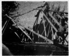
AB28211—The Teco truss, designed by Timber Engineering Co., Washington, D. C., permits clear span roof construction on residential housing projects, both single unit and multiple. It is adaptable to most architectural styles from low pitched ranch style roofs to steeper slopes of Colonial and Cape Cod. Savings in lumber compared to conventional joist and rafter construction vary from 15 per cent to more than 30 per cent in long spans.
