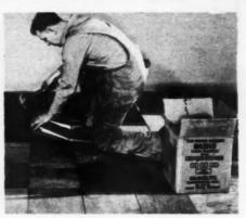
AB28232—Hasco block flooring is a prefabricated, pre-finished flooring of balanced construction that has little or no expansion or contraction. Product of the Haskelite Manufacturing Co., Grand Rapids, Mich., it can be layed in mastic right on a concrete sub floor or layed in any modern home. The 12-inch by 12-inch size fits architectural specifications and achieves a pattern of pleasing appearance. Red Oak is the material used for construction.
