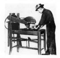
blade cover; streamlined positions for instant one-man change, and adjustable conveyor clamps, both elevating and non-elevating types. This model also cuts intricate shapes without stops for adjustments. It is produced by Clipper Manufacturing Co., 2800 Warwick, Kansas City 8, Mo.
