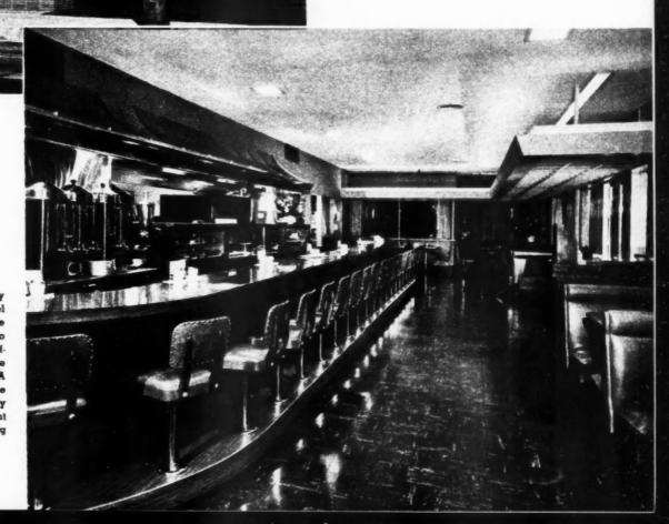
RIGHT: Copper canopy above, and stainless steel panels on each side of the pass window leading to grill area, provides an effective background for the counter arrangement. A feature of the interior is the egg crate design canopy that diffuses the fluorescent lighting from the ceiling
