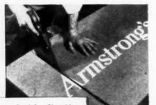
Saw into Temlok Sheathing anywhere; you'll find the same brown color. That's asphalt. It waterproofs every fiber, yet doesn't gum the saw. The picture at right shows some of the first pieces of Armstrong's new Temlok Sheathing being erected in a test panel. First tests show Temlok has a high margin of extra strength and ability to take rough handling.
