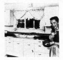
corners where back splash meets the flat top. The floor cabinets are bolted together and the tops joined with a watertight seal, giving a one-piece custom-built effect. This method of fitting tops makes the joints waterproof, greaseproof and dirtproof. Developed by the Midwest Manufacturing Co., Galesburg, Ill., this top is identified as their Kustomized Top.
