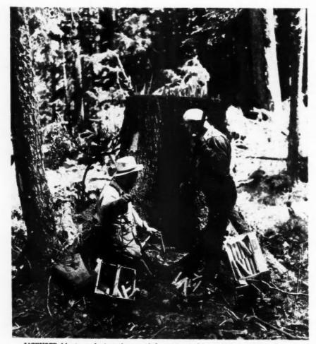
LICENSED blasters placing charge of dynamite at base of stump preparatory to blasting it loose, as one of first steps in removing it from Wedgwood Rock tract
