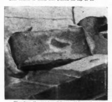
Therefore the mortar did not stick to the top brick. A good bond was not secured.
