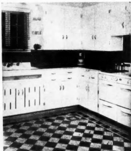
THIS kitchen combines Flexi-Floor and Wall-Flex, products of R.C.A. Rubber Co.
