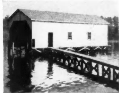
MOISTURE-RESISTANT . . . decades of weather and wet atmosphere will leave this Apac-clad bathhouse safe and sound.
