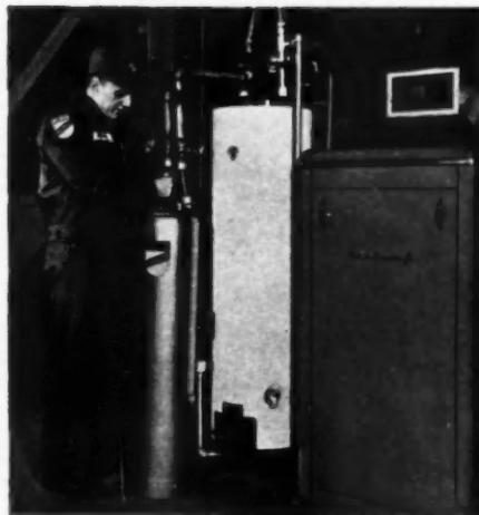
CULLIGAN's water softener is installed in water line. Culligan's soft water service is available in most hard water areas
