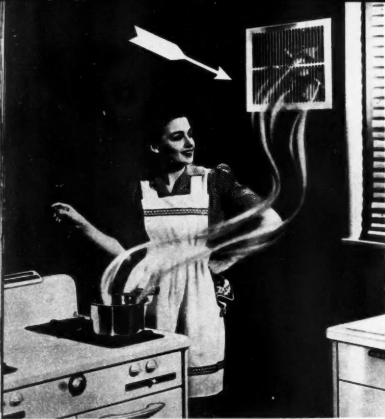
IF kitchen range cannot be installed against an outside wall, it should be close to one. This ILG photo shows vent fan action
