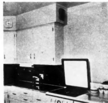
STEWART Manufacturing Co. unit is put at end of soffit above range. This type is used when range is against inside wall
