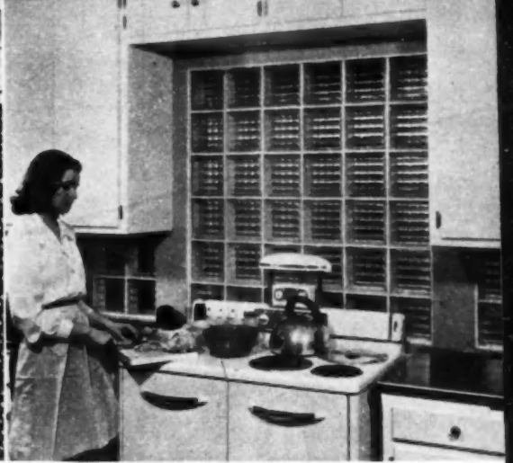
ADDITIONAL light is obtained with Insulux glass blocks over the work area
