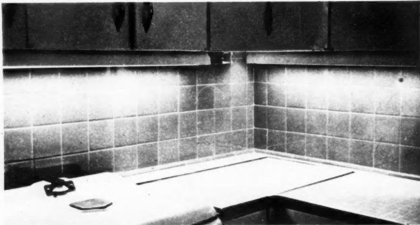
THE CERAMIC-TILED work surface to right of the washing machine forms the cover for a tile-lined clothes hamper. Ceramic tile was also used here for the backsplash
