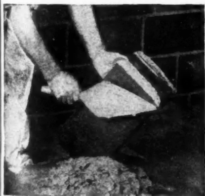
Method 1. Full head joints should be thrown onto both edges of the block to be placed, or—
