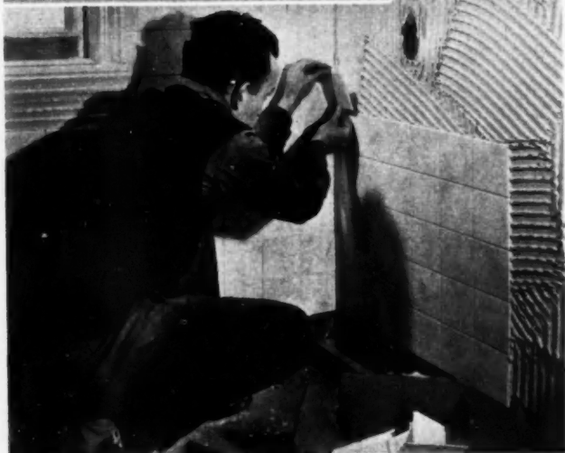
FOUR basic steps in application—smoothing the wall; leveling; plumbing, and applying
