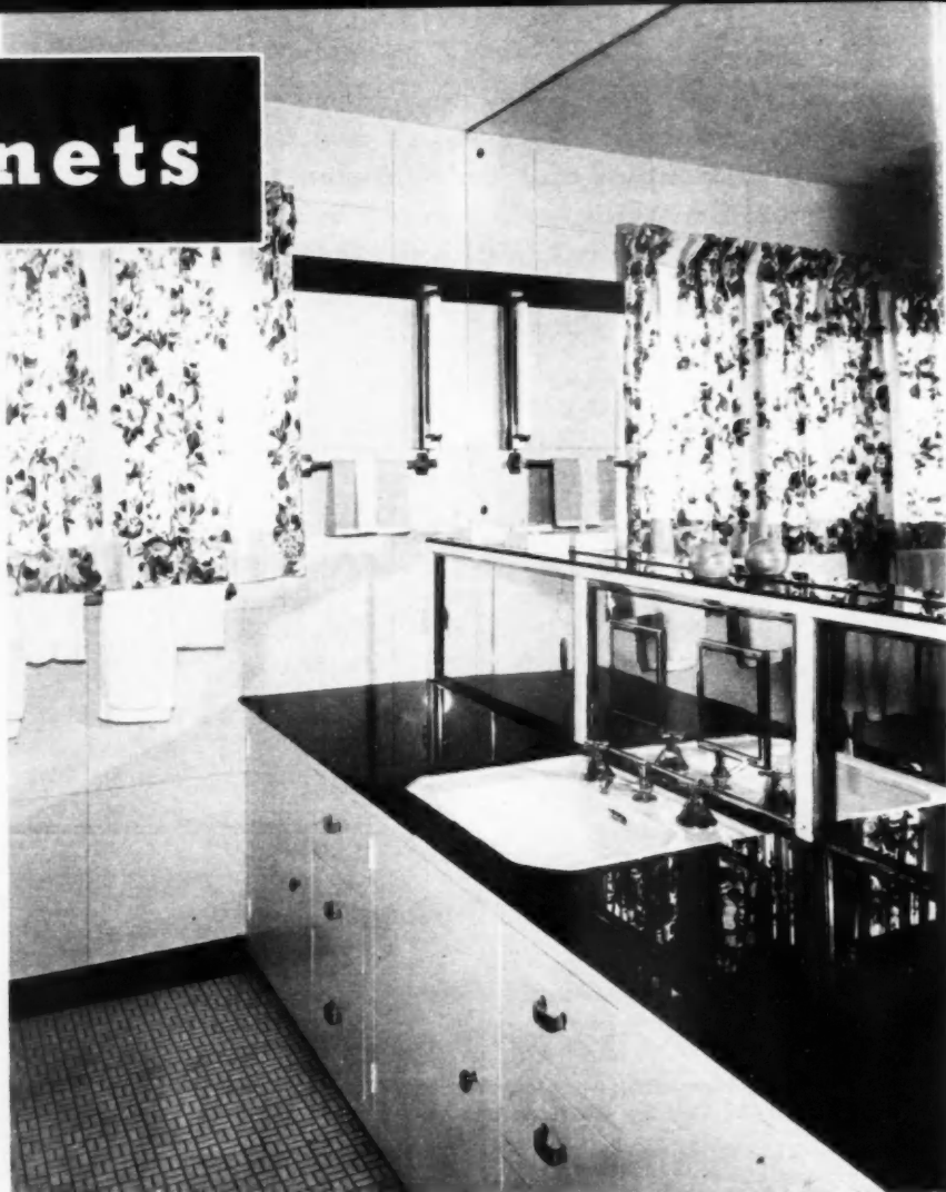
BATHROOM is almost walled-in with glass. Colored Vitrolite used with wood cabinets
