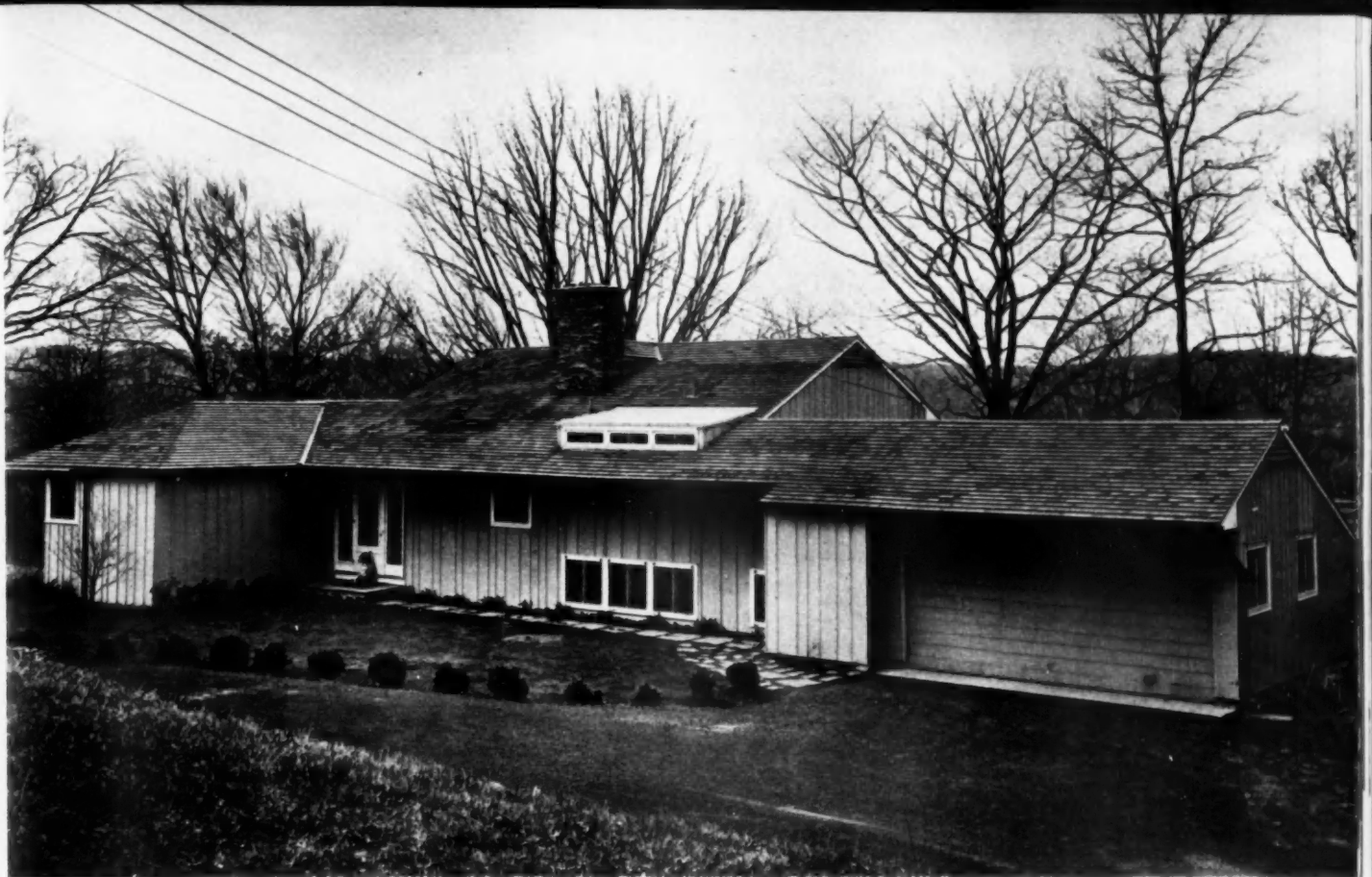
WESTERN pine siding with battens gives vertical accent to this horizontal ranch-style, three-level design
