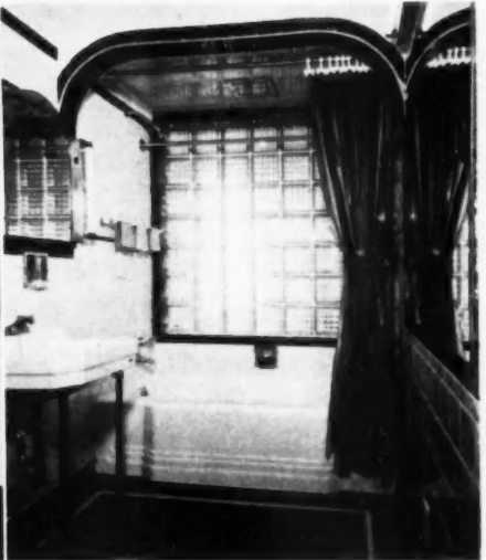
STYRON plastic tiles on walls, arch and ceiling. Dow Chemical Co., Midland, Mich.
