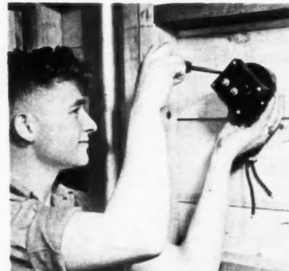
THIS is type of small transformer which provides low voltage required to operate the new remote-control wiring system
