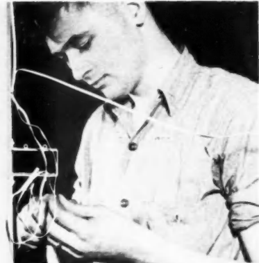
FLAMENOL-INSULATED wire of small size carrying 25 volts is installed in accepted manner without any further protection
