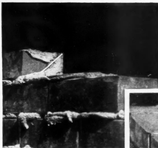
Nail holes frequently connect with voids in the head joints which in turn connect with unfilled furrows in the bed joint.
