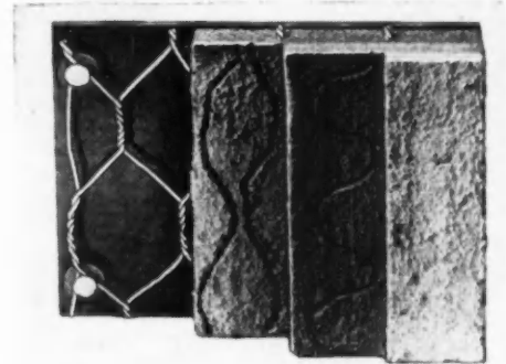
Sectional view of finished wall. Each strand of Keymesh reinforcing is completely imbedded by the scratch coat.
