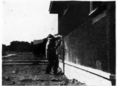
Keymesh being applied to side of house. Note how it unrolls flat—no bulging or sagging.
