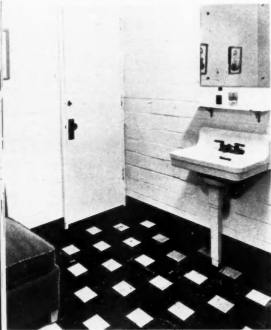
INSTALLATION of marbled rubber tile floor. Fremont Rubber Co., Fremont, Ohio
