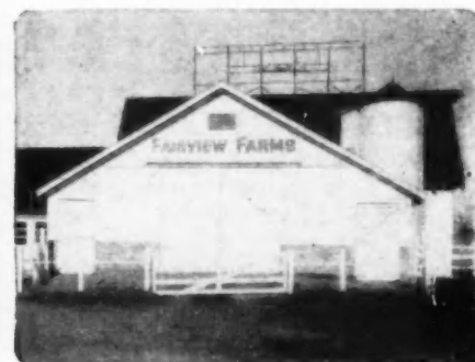
6. Stock barns, silos and other farm structures subject to high humidity.
