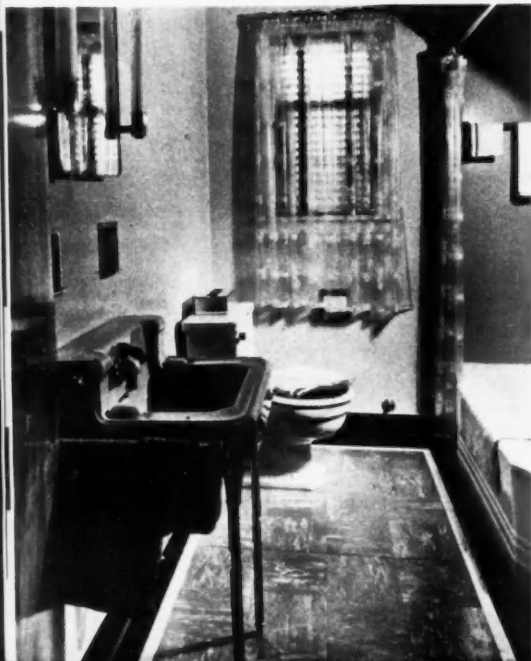
HAKO asphalt tile is used over concrete; moisture proof. Made by Hachmeister Inc.
