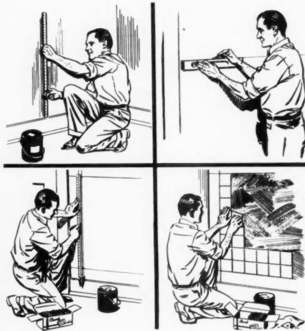
FOUR basic steps in application—smoothing the wall; leveling; plumbing, and applying
