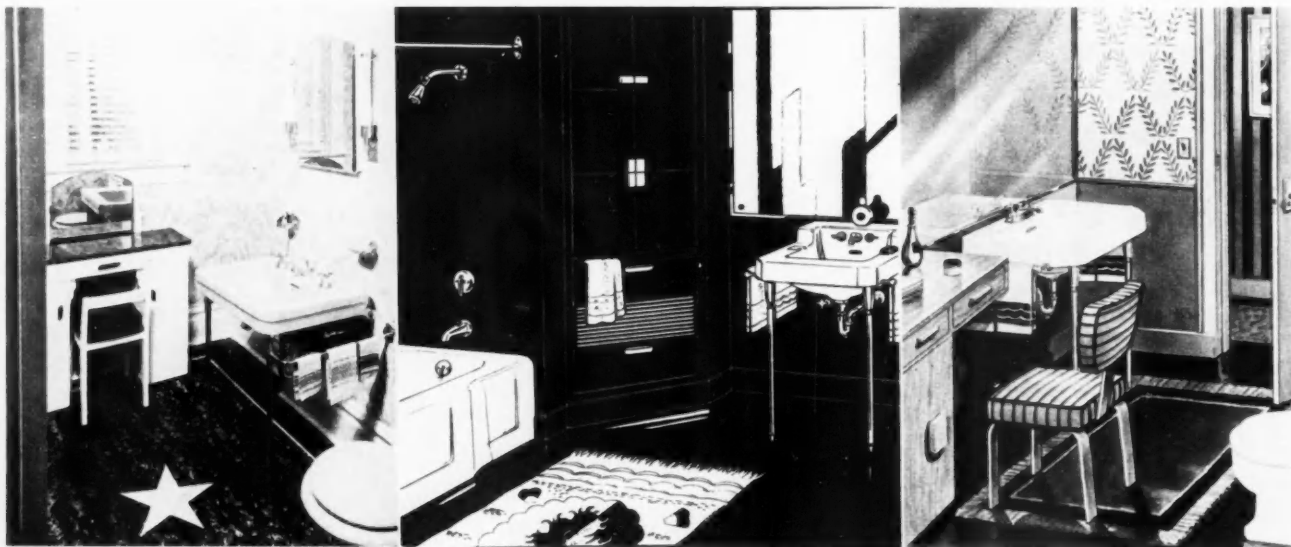
BATHROOM installations. Storage provided by built-in cabinets. Fixtures at left by Plumbing and Heating Industries Bureau
