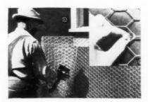
force stucco. It is available in two weights, woven of 17-gauge galvanized wire into a 1½-inch hexagonal mesh, and 18-gauge galvanized wire in 1-inch mesh.
