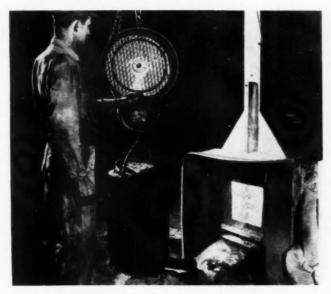
2 BACKGROUND colors are prepared on the floor above mixing machines and poured through hopper openings
