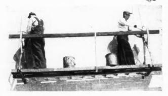
Faster, easier, safer operation of suspended scaffolds is provided by this new SAF-T-SWING winch and stirrup unit. A complete SAF-T-SWING Stage includes two winches—each with attached stirrup and 150 ft. of steel cable—guard rail and center post. The stirrup can also be replaced by a bosun's chair.
