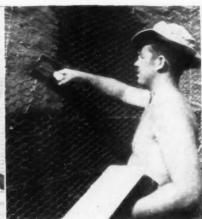
PLASTERER applying scratch coat
