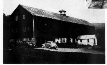
HUMIDITIES in barn ranged from 82 per cent to 91 per cent during tests. In insulated, ventilated barn, variation was 72 to 84 per cent—proper herd conditions
