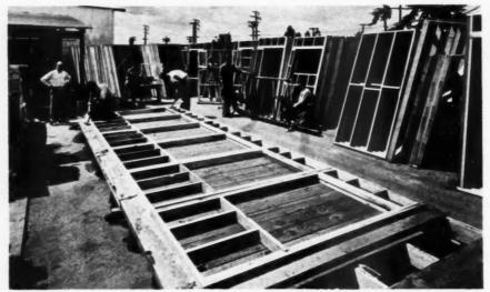
ALLIED Building Supply Co. yard, showing jig table and stock of completed wall panels
