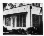
new use for the Plexiglas material. The shutters of the jalousies will not crack, warp or check, even after prolonged exposure to sun and weather, because of the durability of the material from which they are made. They are extremely light in weight. Colors can be selected for any decorative scheme, or translucent white can be used where privacy is desired. The jalousies serve as awnings or storm shutters.
