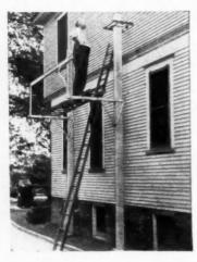
bering. The scaffold may be adjusted to any working height without loss of excess time. Since only ½-inch lag screws are needed to hold the scaffold support in place, surface of the construction being worked on will not be marred. The Wetzel Scaffold is especially suited to remodeling work, or for scaffolding in halls, auditoriums, and gymnasiums.
