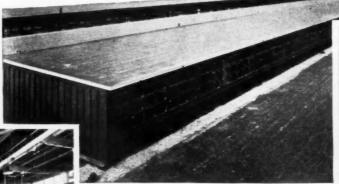
A view of the Truscon Ferrobord Steeldeck Roof, the permanent answer to roof problems. Ferrobord is formed of either 18 or 20 gauge copper bearing or electrogalvanized strip steel with interlocking members. Truscon Ferrobord Steeldeck Roof provides a smooth, quickly installed, fire-resistant surface over which any type of built-up roofing can be applied, with or without insulation.
