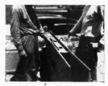
LIGHTWEIGHT interlocking metal members, with clips, holds side board panels
