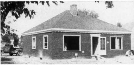
KEYMESH REINFORCEMENT applied on five-room house ready for first coat of stucco
