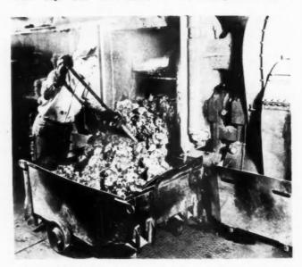
MOTTLE colors for marbleizing are added to the mix a short time before the mixing cycle is completed
