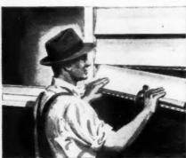
first of all - forget about waves buckles with Kaiser Aluminum Siding! It has a pre-formed curved surface! As each piece is nailed down, the curve produces a rigid surface tension which eliminates distortion.
