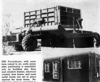
and window frames, electrical conduit, fuse boxes, and room outlet boxes are set in place against the inner forms. Reinforcing steel is mounted to complete the preparation for placement of the outer forms layer, four sets of house for LeTourneau Tournamixers
