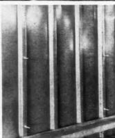
Where metal sidewalls were required Truscon Ferroplate Siding was used throughout the building. Used alone or in conjunction with brick, Ferroplate offers the advantages of quick construction, fire resistance and economy. Write for literature.
