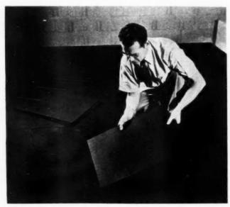
8 INDUSTRIAL tile is hand set, block by block in fastsetting cement. Floors are ready for immediate use
