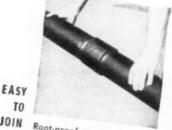
Root-proof, machine tapered joints require no packing.
