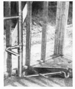
Drainage installation of Chase Copper Tube in one of the 280 homes built by Levitt & Sons, Strathmore at Roslyn; L. I. Distributor: Gar Supply Corporation, Long Island City, N. Y.
