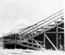
2. Ground moisture and rain held in joints, etc., of outdoor structures.
