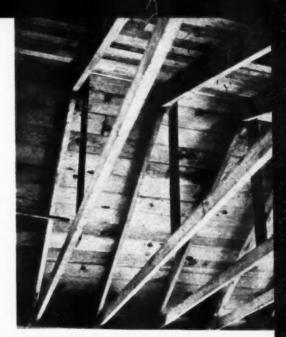
ROOF trusses for 16-foot span are fabricated on ground, raised in position
