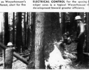
IT TAKES SKILL to drop a big tree in exactly the right spot, without need lessly breaking or wasting timber. The power saw being used by these Weyerhaeuser fallers adds ease and certainty in this ticklish job.
