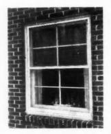
cause they mount close to the basic window. Because narrow-rolled 52S aluminum is used in the frames, they are thin enough to allow for screen or sash storage when not in use. A flat screw-type lock makes draft-free ventilation possible by holding the lower sash in any desired position. (Continued to page 176) 1948.
