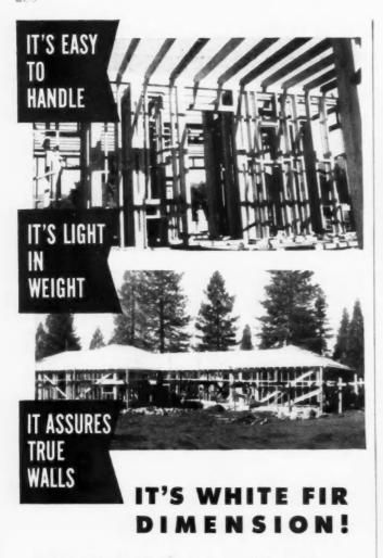
Wide-awake builders, architects and dealers are today taking advantage of the superior characteristics of White Fir dimension for framing purposes. Because of its straight grain, White Fir studding provides a true wall for plaster base and White Fir floor or ceiling joists assure a level surface for floors.
