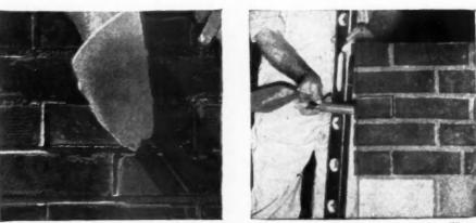
Realignment of a brick should not be attempted after a higher or following course has been laid. When a brick is hammered back into line, the bond between the brick and mortar is broken. Cracks due to such realignment are frequently found at the corners of the wall.
