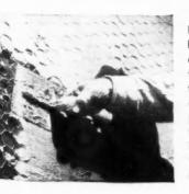
Plastererslike Keymesh because the surface' is smooth to the trowel in any direction. Keeps its proper distance from the backing, insuring a "true" wall of even thickness,
