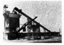
THIS huge batching plant at Park Forest project will mix 650 yards of concrete a day. Sand and gravel are dumped directly from freight cars into a pit and carried on moving belt to the mixer
