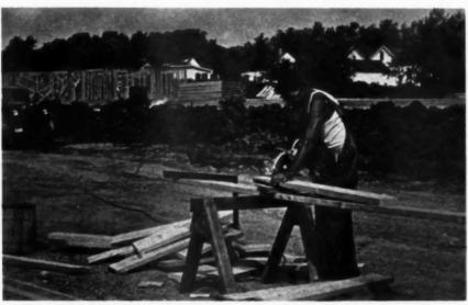
POWER saws, with power supplied from generator mounted on truck, were used anywhere on the site they were needed. The men worked in specialized crews
