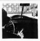
A829226—Remote radio control for power operators on upward acting residential garage doors. Crawford Door Co., Detroit, Mich. Driver presses button on dash when approaching driveway. Marvel-lift door opens, yard and garage lights go on at touch.
