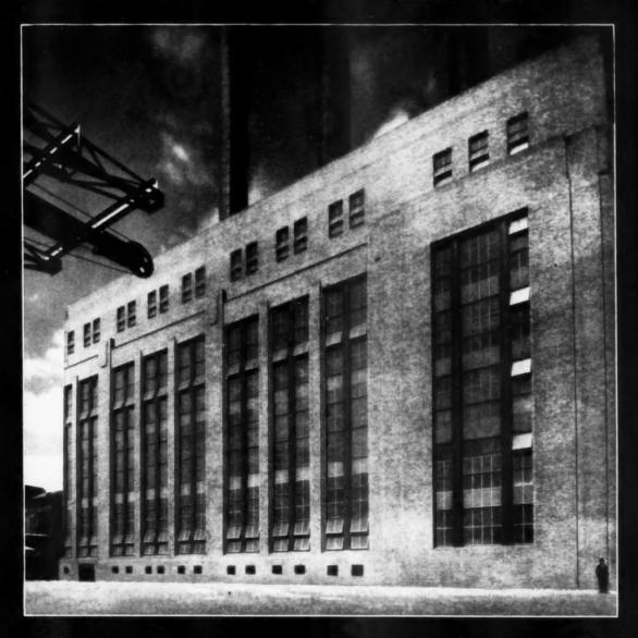
THE HOPE'S LOK'D BAR FACTORY SASH recently installed in this Power Station building are made to special size and layout. Their height, 63', 0", is indicated by the size of the figure in the lower right foreground. The mullions are 10 gauge pressed steel reinforced by structural members. Hope's LOK'D BAR Catalog describes, with full-scale drawings, the exclusive principle of their design, and Hope's Engineering Department will be glad to submit details for similar installations on request.
