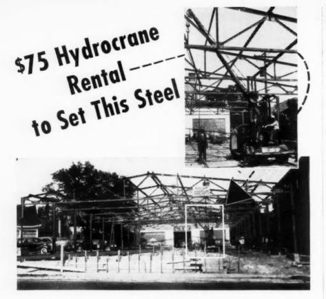
In just one day — including two miles of travel to and from job plus unloading steel from trucks — a Bucyrus-Erie Model H-2 Hydrocrane set this 60' x 140' steel structure — picked up 50-foot steel trusses weighing  $1\frac{1}{2}$  tons and placed them in position 24 feet above the ground. The contractor rented the Hydrocrane for only \$75 including operator's pay and gasoline cost.
