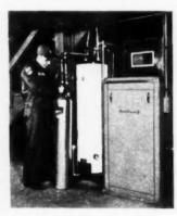
AB29106—Culligan soft water service unit. Culligan Zeolite Co., Northbrook, all. Soft water available on a service basis. Unit is installed to supply water in home. Exchanged by company service man at regular intervals for another unit of freshly regenerated zeolite. A monthly charge made for service.
