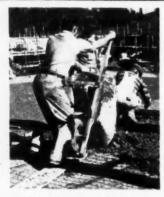
AB29196 — Pittsburgh Steeltex for floor lath. Pittsburgh Steel Prod-ucts Co., Pittsburgh, Pa. Offers structural advantages and economies in light-slab concrete floor and roof construction. Gives maximum reinforcing value and facilitates reinforcing value and facilitates proper curing of concrete through maintenance of water-cement ratio.
