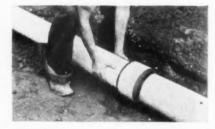
WIPE END of next length of pipe and apply primer; then insert this length with twisting motion into coupling
