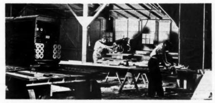
TWO LARGE portable generators on trucks were used to run total of 18 power saws. At this shop, centrally located in Sunset Park, precutting made greatest time-saving
