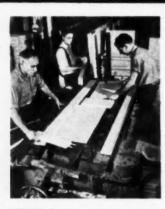
AB29107—Prespine panels. Curtis Companies, Inc., Clinton, Iowa. Door panels are cut and machined just like wood. Composed of sawdust mixed with a chemical compound, it comes out of heat press in large sheets resembling in color the natural wood. Material is used for all doors and kitchen cabinet panels.
