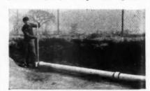
GOING to other end of length, push it into place with rod and block of wood. Repeat procedure starting with step one
