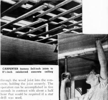
through the wood joist into the concrete, holding the joist securely. The operation can be accomplished in five seconds in contrast with about a half hour that would be required if a star
