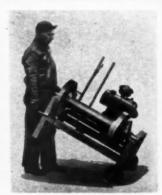
AB2973—Portable hoist. King Manufacturing Co., Chicago, III. Produced in four models, they are light enough in weight to be loaded and unloaded without difficulty. Handles like a barrel or bag truck. Are ruggedly built, compact, and easy to operate. Supplied with an air-cooled motor, economical and easy to run.
