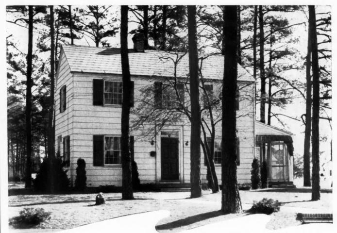
Note the attractive appearance of this suburban home protected with #57 "Century" Asbestos-Cement Siding and #30 "Century" Side Lap Roofing Shingles.
