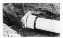
PUSH coupling over pipe with twisting motion. Then using rod and block of wood, push coupling firmly into position
