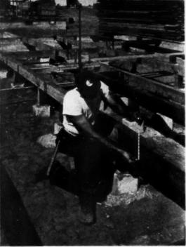
THE 4x6 girders and the 2x6 t6g subflooring used on this job are chemically treated as insurance against termites
