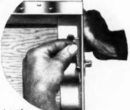
2 Drop Tie Key into the Loop. This locks the UNI-FORM and Tie into one integral unit.
