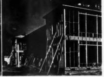
EVEN THOUGH climate is mild, framing for both one and two-story dwellings is of exceptionally good material, well braced. Basements are rarely included in this section
