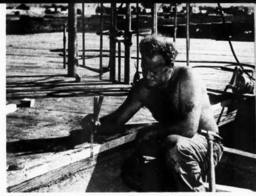
ONE BUILDER uses tongue and groove 2x6 sub-flooring over 4x6 girders for his floors
