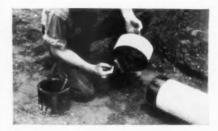
AFTER cleaning end of pipe and inside of coupling with dry cloth, apply primer to both the pipe and the coupling
