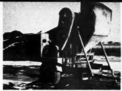
POWER wheelbarrow is popular with laborers, builder reports. Scoopmobile speeds handling of foundation excavation and loading of other earth material. Large concrete mixer, two jeeps also are used
