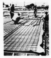
AB29165—Waterproof reinforced paper named Sisalkraft. The Sisalkraft Co., Chicago 6, III. Applied over fill in radiant heated floor job, as illustrated, it prevents small fingers of concrete from dropping down into the fill. These fingers carry moisture and cold up from ground into the concrete. Sisalkraft protects floor.
