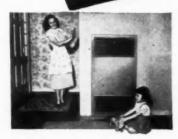
WALL FURNACE—Registers on both sides of the partition. 42,000 BTU. Output.
