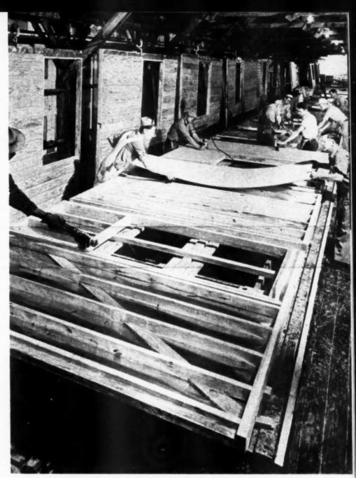
ONE of the production lines in the Crawford Corporation plant at Baton Rouge, La. Here men do specialized tasks in assembling precision-cut lumber and other parts into complete wall sections for the houses
