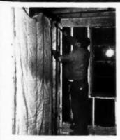
A829215—Cellulite cotton insulation for soundproofing. The Gilman Brothers Co., Gilman, Conn., Produced in blankets for use as sound deadener. Installation simple. Blankets are hung by weaving in and out between studs. In a staggered-stud fest wall, 3-inch Type E Cellulite cut passage of sound to whisper.
