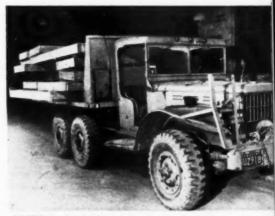
SEVEN 6-wheel drive trucks with winches are used to transport finished sections of houses from the plant to job site
