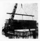
AB29360 — Bulldog concrete forms. Bulldog Concrete Forms, Inc., New York, N.Y. Basic form, 2x4 feet steel panel, set horizontally or vertically to assemble pattern of footing, tie beam, column or other structure. Wide variety of other widths available.
