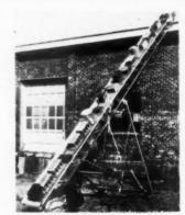
A829143—Mulkey Portable Elevator. Sam Mulkey Co., Kansas City, Mo. Manufactured in four sizes. Easily maneuvered and placed in position. Adjustable to accommodate extensions. Balancing permits one man to handle and operate. Can be used for transporting all kinds of building materials. Savings in labor cut costs.
