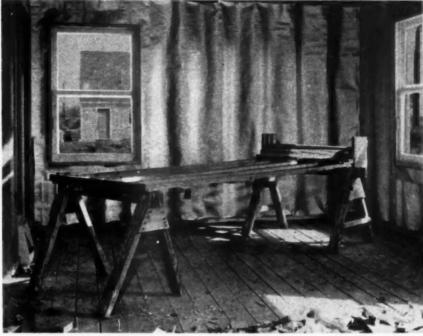
IIG, made at on-site shop, is used to speed up application of special sheathinginsulation material. Exact lengths of the material can be quickly cut, without necessity of measuring. Material feeds across jig table from roll on one end
