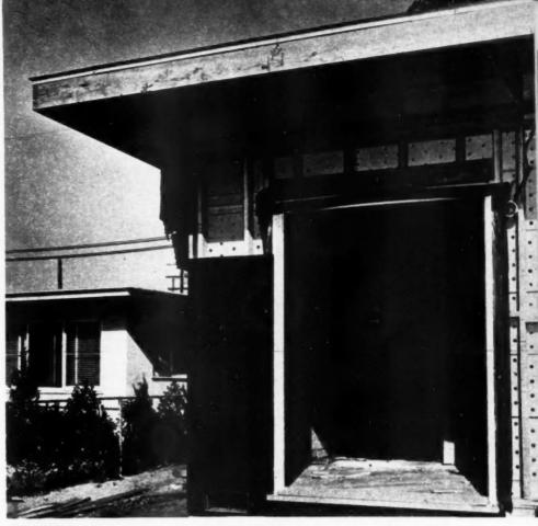
SHEATHING is rarely used on houses in California. Stucco is a popular exterior finish and is applied directly to stude over felt paper and chicken wire for reinforcing
