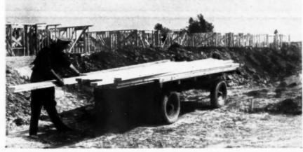
SMALL trailers saved costly tie-up of trucks. Load of materials can be left in front of house where needed until trailer is empty, then one truck can pull trailers back
