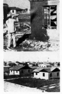
SPRAYING cement on exterior walls with let-Crete girgun is done in low-cost housing by Farmers Construction Co. Wall partitions are of Texcrete blocks
