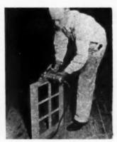
AB29181 — Stanley-Carter "Wasp" Power Plane. Stanley Tools, New Britain, Conn. An electric plane with patented spiral cutter which produces smooth waveless surface. By substituting shaper cutters, it becomes a miniature planing mill and will make surface beads, tongue and groove, and other moulding cuts.
