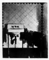
AB29142—Aluminum wall tile. Metal Tile Products, Inc., Hastings, Mich. "Alumitile" made in a variety of shapes and sizes in 14 colors. Special finish is highly resistant to household acids. Easily applied to any smooth wall surface with a special waterproof mastic. Special process assures a good control of all color.
