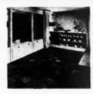
AB29256—Hasko block flooring. Haskelite Manufacturing Corp., Grand Rapids, Mich. Mutiple plies of veneers cross-grained to produce block 12 inches square by 36-inch thick, of Northern oak. Tongue and groove. Applied over concrete or wood.
