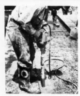
AB29377—Newest addition to the Mall vibrating line. Mall Tool Co., Chicago, III. A universal electric motor-driven, one-man vibrator for use in tight spots. Will place concrete fast and efficiently with a minimum of operator effort. The complete line of Mall power tools are subject of booklet offered free.
