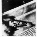
AB2976 — Tub-Tite caulking compound. The American Fluresit Co., Cincinnati, Ohio. A resin-based plastic caulking applied direct from tube, then smoothed with applicator. Tub-Tite dries within an hour. It remains flexible, expands, contracts with joint.
