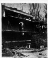
AB29168—New mason scaffold. Requires but one man per jack to install. Height is adjustable in 4-inch steps and manufacturer claims it is not necessary to level ground or bask-fill. Equipment has been tested and received Industrial Commissions approval in several states. Wilson-Albrecht Co., Minneapolis, Minn.
