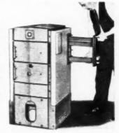
AB29188—Herewith the latest addition to the Smith-Mills residential boiler series. H. B. Smith Co., Inc., Westfield, Mass. Known as No. 1500 Smith-Mills boiler. Is furnished jacketed and complete with a built-in tankless heater that supplies hot water instantly to fixtures. Boiler is finished in cream and black.
