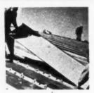
AB29265—Monel sheet for roofing. The International Nickel Co., Inc. New York, N. Y. May be cut, formed, joined and soldered into standard roofing parts with regular tools and methods. Nickel-Copper, .018-inch thick, corrosion-resistant.
