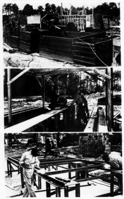
COMPLETED WALL sections ready for site assembly are shown above. When necessary, power machine illustrated trims joists to length on site. Accurately sized nailable steel stude are welded into wall sections at project
