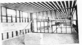
Interior view of school under construction. Note how wood collateral is nailed directly to metal framing.
