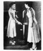
any furnace flue six inches or larger. By means of grate baffle, draft is induced through top causing down-draft which dries and super-charges the burning of the contents. Finished in brown bronze, unit measures 23 inches in diameter, 32 inches in height. Burns wet or dry garbage. Majestic Co., Huntington, Ind.
