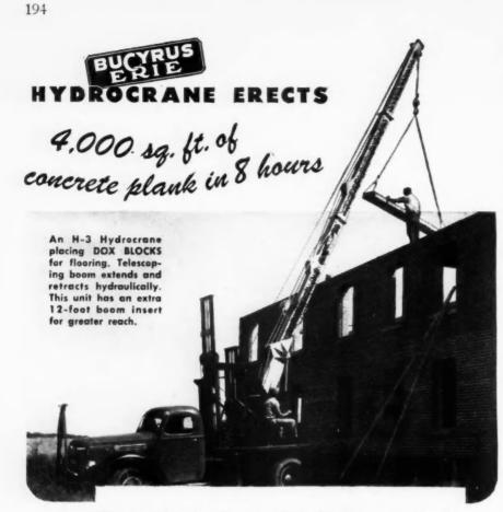
**B**Y USING a Bucyrus-Erie Hydrocrane, Vander Heyden, Inc., Milwaukee, Wis., building contractors, erected 4000 sq. ft. of their prefabricated DOX BLOCKS concrete planking in 8 hours. On average jobs they place from 2000 to 3000 sq. ft. per day, mostly floors and ceilings for housing and commercial building.
