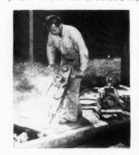
volt tools and floodlights. Breaker and generator make compact combination that can fit in trunk of car and can be put into operation quickly by one man. Breaker is unaffected by dust or abrasive particles. Motor has no brushes or commutator. The Homelite Corp., Port Chester, N. Y.
