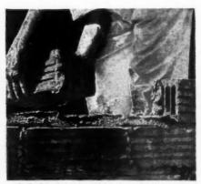
Method 2. A full head joint should be thrown onto he edge of the tile in place and also onto the opposite edge of the tile to be placed.
