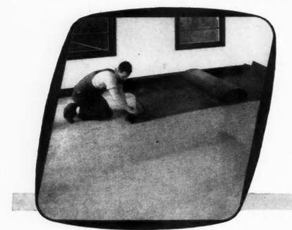
PLYBASE is a NEW GRADE of Interior-type Douglas fir plywood with a face of B (solid) veneer, and a back of D veneer. All sanded both sides. For full details on PlyBase use and application, see Sweet's File, Architectural, or send for the new 1949 Basic Plywood Catalog. Write the Douglas Fir Plywood Association office nearest you: Tacoma Bldg., Tacoma 2, Wash.; 1707 Daily News Bldg., Chicago 6; 1232 Shoreham Bldg., Washington 5, D. C.; The 500 Fifth Avenue Bldg., New York City 18.
