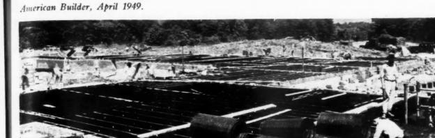
WHEN JOISTS are in place they are connected with steel bridging strips. Fiber backed steel mesh is nailed to steel joists as base for the concrete slab
