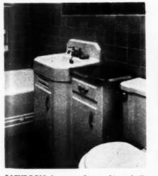
BATHROOM lavatory has cabinet built around it to provide additional storage
