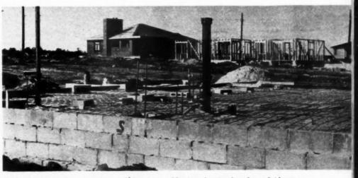
TYPICAL foundation of a Diamond Bar home. Moisture barrier has been laid over which steel reinforcing has been placed ready for concrete floor slab to be poured
