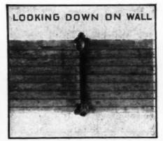
Enough mortar should be used to cause excess mortar to coze out of the joints on both sides of the tile.
