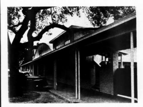
STRUCTURES in rear of arcade are of concrete block. Attractive canopy extends out 10 feet
