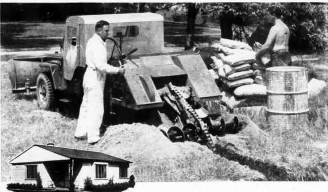
This two bedroom house requires a trench 35' by 31' and 42" deep for a concrete footing. The Jeep-A-Trench does the excavating in 3 hours—a saving of 32 man hours over ordinary digging methods. After trench is completed, boom is raised to transport position and the unit is ready to move to the next job in a hurry.
