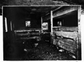
HERE is the interior of the old hog house after remodeling. Note dry condition of floor, ventilating duct and adequate insulation
