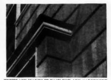
TEMPLATE MAKES IT EASY FOR ANY CARPENTER TO OBTAIN A TIGHT, CLEAN CORNER FIT
