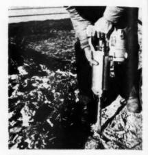
SYNTRON hammer used for breaking up concrete or rock is easily handled
