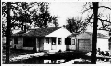
SIMPLIFIED construction is evidenced in the shed roof design as applied to the "A" house with attached breezeway and garage
