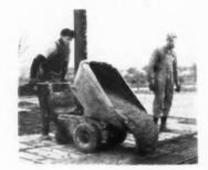
foot pedal. Equipped with a 9 square-foot steel platform, it hauls half-ton loads. Powered by enclosed engine, climbs 20 per cent grade fully loaded. Three gallons of fuel provide 8 hours' continuous service Bell Aircraft Corp., P.O. Box IAB3, Buffalo 5, N.Y.
