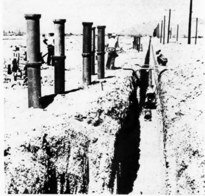
MORE than 11,000 feet of 8 and 10-inch vitrified clay pipe go to provide sewerage facilities for the first 700 homes. Over 50 miles of pipe will be installed
