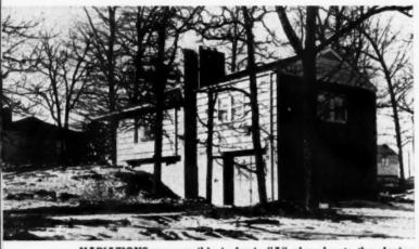
VARIATIONS are possible in basic "A" plan due to the sloping terrain. Exposed portion of basement provides room for garage
