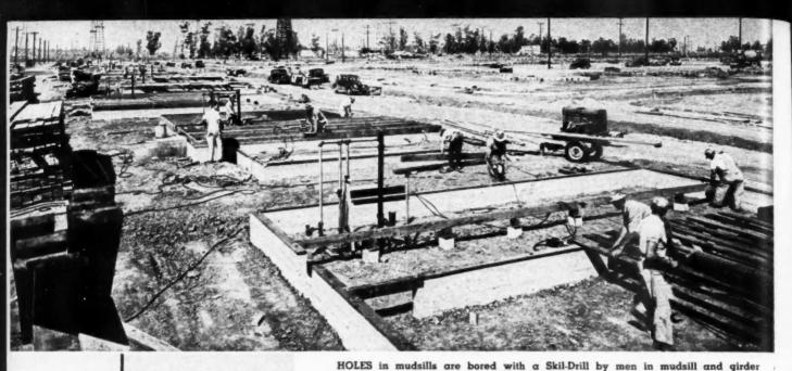
crew. Left, a Cleveland trencher digs foundation footings. By careful stripping, oiling and handling, foundation forms have been used more than a hundred times
