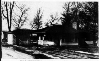
TWO BEDROOM house takes on a different appearance through the application of a hip roof, breezeway, and attached garage
