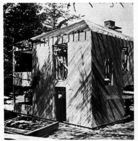
CONVENTIONAL wood sheathing secured diagonally to wall stude for rigidity
