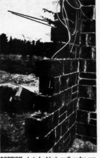
PORTION of cinder-block wall under construction. For additional rigidity reinforcing rods are placed in blocks. Voids in blocks are used for extending conduit
