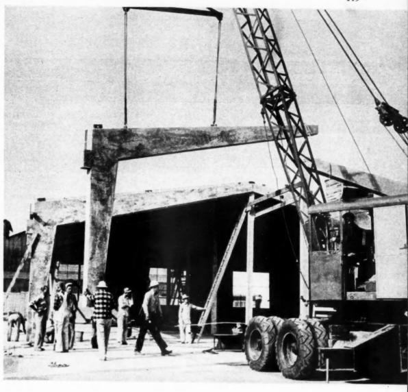
IN ANOTHER Buttress and McClellan project. truss is aligned by crew experienced in tilt-up method. Operations are planned by a unified staff of architects, designers and engineers, specialists in the system
