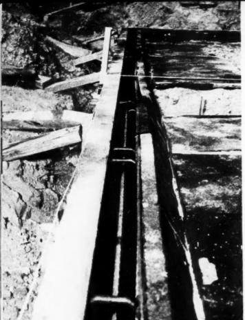
METAL pieces are placed to hold forms in position until combination walls and footings are poured. Afterwards. pieces will be removed. Footings and walls rest on 12-inch piers that are spaced about 5 feet 9 inches apart
