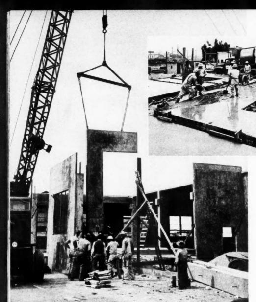
CASTING of wall on concrete floor. This step is followed by trowel-finishing, after which panel is hoisted in place
