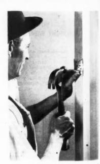
It is so simple! Nail Fasteners to stude in new construction. Fastener prongs enter back of panel and clinch.
