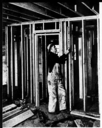
AN example of a typical wood stud bearing partition in a frame house. This is a type most frequently used
