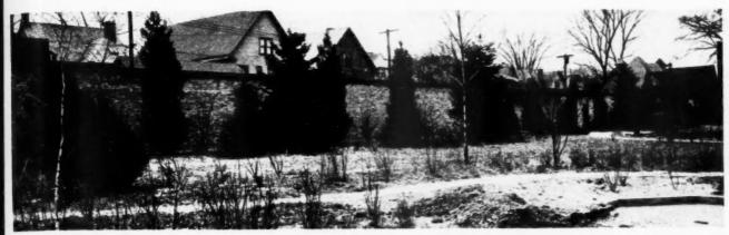
STRUCTURE, which resembles brick garden fence, houses 65 automobiles. Construction is steel and masonry. Extra precaution against damages from fire is installation of fire fighting equipment
