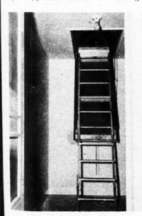
DISAPPEARING stairway in storage room makes ample space in attic available
