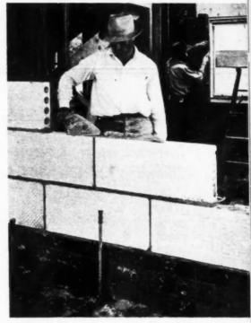
GYPSUM block, brick and similar materials are used with concrete slabs
