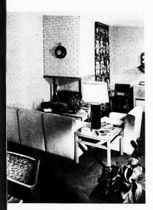
A CORNER in living room. The brick over-mantel of fireplace is extended around entire end wall and a portion of side wall. Fireplace is of open type with 3 inch pipe support at corner, and with hearth raised above floor
