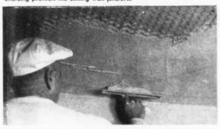
First coat of plaster trowels on quickly and easily over Keymesh, providing an even base for a smooth finished job.
