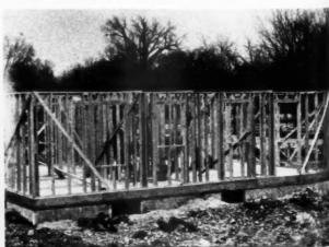
CELOTEX strip is placed between plate and top of foundation wall to eliminate shims. Tilt-up wall construction is used
