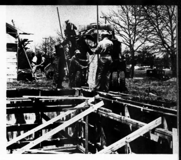
CONCRETE is mixed in transit. Plywood forms are made by the firm, ties and clamps are factory made. Here concrete walls are poured for a group of the company's low-cost homes
