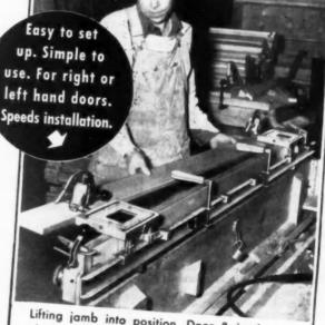
Lifting jamb into position. Door & jamb are clamped together, hinge recesses cut at
