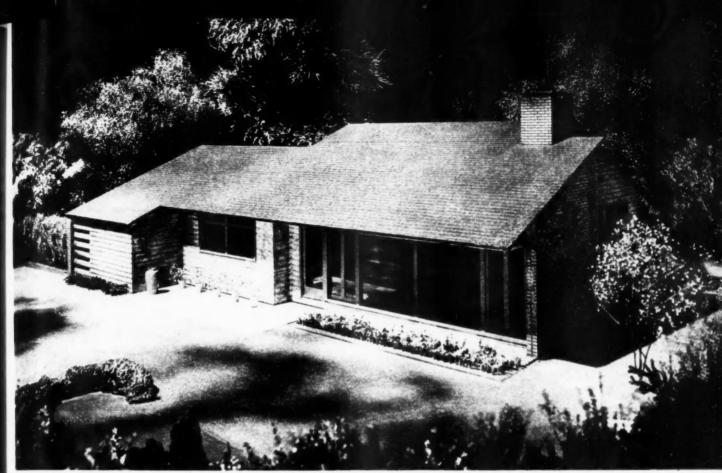
GARDEN view of house. This three dimensional scale model was produced for Servel. Inc., Evansville, Ind. The house is now being built in various sections of the country. It is designed to effect building economies and to enable the individual constructing a medium priced house to obtain air conditioning as inexpensively as a residence with just a heating system. Simple lines feature the house
