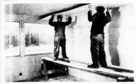
TWO thicknesses of gypsum board being applied, the first layer nailed, the second glued
