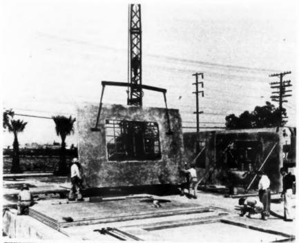
FINISHED panel, complete with sash, is raised to upright position and swung in place
