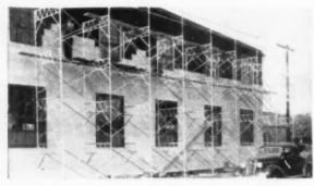
Erection is simple...fast...labor-saving. Each frame slips into place quickly over sprockets in frame below... and locks securely. Available parts include frames of various sizes, braces, guard rails, ladders, trusses, brackets, etc. These can be assembled in any combination to fit the specific needs of the job. Safe, strong, long-lasting "Trouble Saver" Scaffolding saves time, money and labor.
