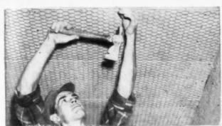
Lathers applying Keymesh Reinforcing to ceiling. Notice how the reinforcing protects the ceiling-wall juncture.
