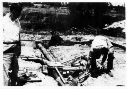
INVERTED blower type oil-fired furnace supplies heat through clay pipe ducts to warm air registers in rooms. Heat loss is exceptionally small, according to Virgil Place
