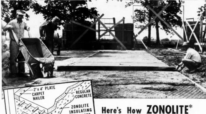
This diagram of a floor with radiant heat coils shows one of the many ways in which Zonolite vermiculite Concrete can be used efficiently.
