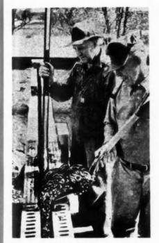
POURING and rodding vermiculite insulating concrete in a 10-inch tile cavity wall
