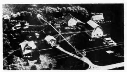
FARM showing overhead wiring to buildings and from the distribution line
