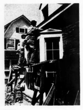
FLASHING is installed over bay window, left, as student's project this year nears completion
