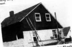
One of the houses in the development, using ES-nails to apply shingles to insulation sheathing.
