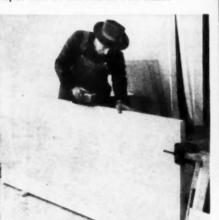
Interior doors are sanded free of all scratches and tool marks with the Century and the treated surfaces rubbed down between coats.
