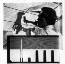
When installing acoustical tile choose a job-designed nail that combines ease of application with these special features: a head end which allows the nail to be driven home without damaging the tiles ... a collar which holds the tiles firmly in place ... annular threading which gives superior holding power. The nails are furnished with a plated finish to prevent rust streaks where moisture is present. Send for free samples and descriptive literature.
