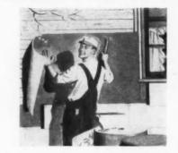
insulate old sidewalls when applying asbestos shingles or other siding, new under-liner has conductivity (k) factor of .25. Reduces wall heat loss up to 24 per cent. Cushions new exterior, reducing possibility of breaking siding during application. Per-mits tight application of shingles, with little chance for siding to rattle in wind when job is completed. Wood Conversion Co., St. Paul, Minn.
