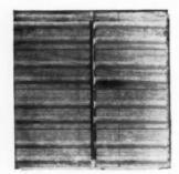
Blocks consist of standard tongue and groove strips bound together by steel splines imbedded in the back.
