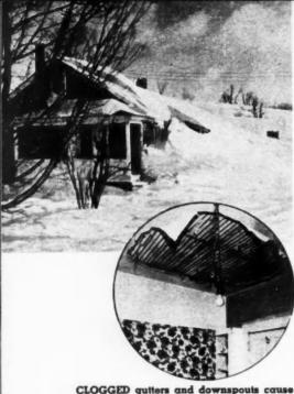
clogged gutters and downspouts cause moisture to back up under shingles and seep into interior; cracked plaster results
