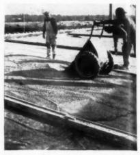
BY laying the insulating concrete in alternate panels, workers were enabled to work alongside the sections being poured
