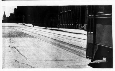
TEN YEARS AGO, in August, 1939, this concrete test paving was laid in Second Avenue North, Minneapolis. The badly scaled section of roadway in the background was made with regular portland cement. The foreground section, laid at the same time, was made with Atlas Duraplastic—the first commercial use of the air-entraining portland cement originated and developed by Universal Atlas.
