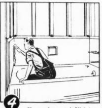
Clean glass and fill joints carefully with the pointing compound supplied. This assures a thorough waterproofing installation.
