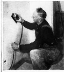
Dry wall taped joints and rough plaster are sanded smoothly and uniformly with the new Century. Ordinarily this type of work runs high in cost because of the time required for the necessarily smooth finish, but the Century, loaded with a 150-grit open coat paper, does it with speed, precision and economy.
