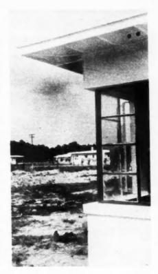
POURED concrete lintel supports corner of roof above this corner window of home in Burkrete subdivision. Remainder of exterior walls are of concrete blocks
