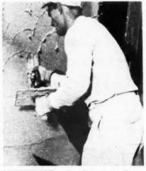
LIGHTWEIGHT perlite plaster is easily applied and provides high sound absorption
