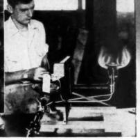
Paul Simon is testing the gas burner for the AS23. Each burner, oil or gas, is completely tested and thoroughly checked. They are checked for fuel leaks, electrical connections and control operation. Not until this careful test is completed and passed is a burner released for shipment with the furnace.
