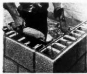
in morter, it forms continuous lateral reinforcing to prevent cracks. Used as reinforcing to tie face brick to back up block, in double wall construction, where insulating dead-air space is formed; for brick and clay tile wall, as well as for reinforcing block walls. Dur-O-Wal Div. of Cedar Rapids Block Co., 656 12th Ave., S. W., Cedar Rapids, Ia.
