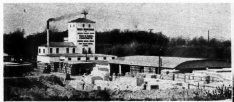
CAPACITY of Hass cement block and brick plant is 5,000 8x8x16 blocks per eight-hour working day. A mix-in-transit concrete service, which company operates in conjunction with plant, right, is the only one of its kind in the South Bend area.
