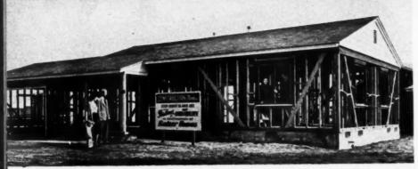
CONSTRUCTION models permit buyers to see how walls, floors and ceilings are built
