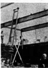
tor moves on wood track which is built by contractor on job site with standard size 2x6 lumber. Steel channel, with all joints electrically welded, provides sturdiness to elevator platform. System may be used in conjunction with any power hoist capable of exerting 400 pound effort on a single line. King Manufacturing Corp., 3146 W. Chicago Ave., Chicago 22, III.
