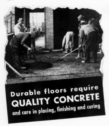
THE PRINCIPLES of good concrete floor construction are simple but vital. Every step is important—the quality of aggregates, amount of water used, proportioning, placing, finishing and proper curing. Strict observance of the principles of quality concrete construction will insure satisfactory floors.
