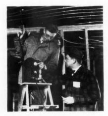
PICK-UP of General Electric leak detector is passed through air surrounding copper tubing of radiant heating system by J. S. Hickey, one of engineers who helped to develop it, William E. Herrmann (right), is engineer in whose home test was made
