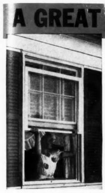
The top storm section slides into position on metal guide strips attached to sides of window frame. Positioning clips hold storm section firmly in top position.
