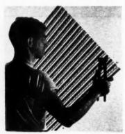
lath is sprayed red; 2.5 pound diamond mesh and 2.75 pound flat riblath are sprayed white, and 4 pound 3/6-inch riblath is sprayed blue. When dealer or contractor receives a shipment, a glance at end of the bundle tells him the weight and type. Lather can easily tell correct position for installation. United States Gypsum Co., 300 W. Adams St., Chicago 6, Ill.
