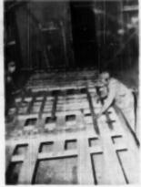
WALL sections, porches and other building parts are produced and assembled in large plant utilizing fast power tools
