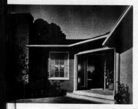
ANGLED wall with lurgecased opening inems a portion of enclosed ports; this provides pretection from inclument wouther for the entrance door. Pull length translucent glass posed admits light; jain entrance hell light; jain entrance hell
