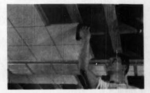
Quick, easy installation. Temlok Tile comes in three convenient sizes 12" x 12", 16" x 16", and 10" x 92", Tiles are simply nailed or stapled along furring strips spaced 12" or 16" on centers over ceiling joists. Lok-Bevel joint provides extrawide nailing flonge which speech nailing or stapling on the job.
