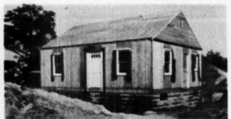
PARTIALLY completed "Fair Deal" panelised house assembled over a full basement. Note plywood sidewalls and road decking with bevel siding on qubic ands. Sidewalls will be completed with wood shingle siding
