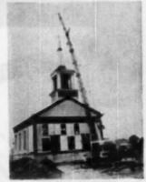
CHUBCH is re-exected at Stratford. Co. after being dismonthed and moved 150 miles with the help of MC-416 Loroin crane
