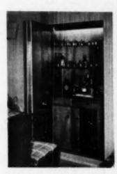
OPEN bur shows the interior finished in surhogenry plywood including the inside iers of felding doors. Ginza shalves above and cuphosends helow provide emple storone and of the counter. Pluorescent light above turns on when doors are opened; exterior face of doors in finished to conform with the officining wood wells
