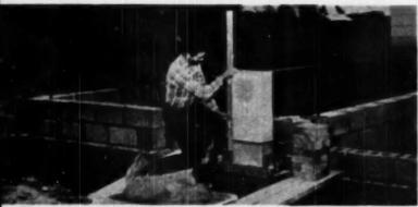
TO ensure a straight, amonth-jointed lining, each successive length at lining tile should be positioned first and the supporting brick work built around it. Too often this is not the prevailing practice. In most cases the brick work is built up first and then the lining is dropped into position inside. The inevitable result is failure to get tight joint between the sections and failure to properly fill apares between lining and brick work
