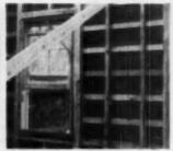
WALL panels illustrating 2x4's dadosawed for receiving 1x3 horizontal wood notling bane strips are shown here. Interier walls are of dry wall type using either paper or point covering
