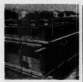
FOOTER terms for foundation walls are leveled accurately,  $4' \times 9' \times \%$ , inch-thirft plywood terms are numbered for re-use without delay. Double 2 x 4 waters, somety's and beauting hold forms straight
