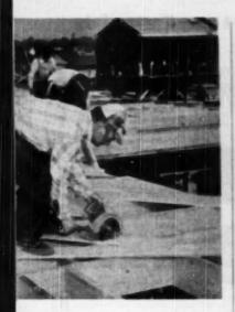
building, and the work they are doing, is coordinated closely with the progress of the radial saws. When outside walls are all cut, and assembly begins, these saws are cutting inside partition members. Plumbing openings and plaster grounds are all provided for so that when the framing crew leaves they do not have to go back to rough these in.
