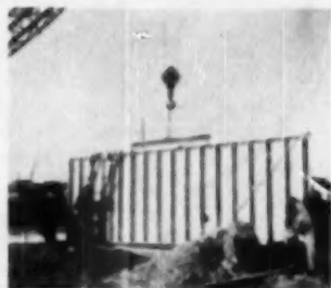
FULL-LENGTH wall panel being guided into place. A light crane facilitates the operation.
