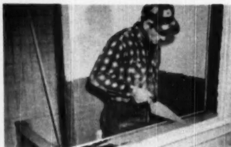
SECOND, apply mortar to sill. Use 1/4 inch thick mortar joints
