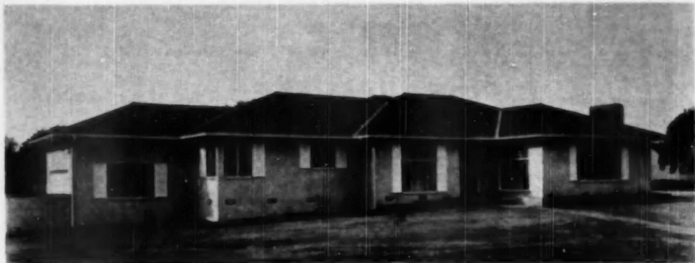
THIS house of 1780 square feet is evidence of Robert Olin's building abilities, but its "extras" are what attract a growing clientele
