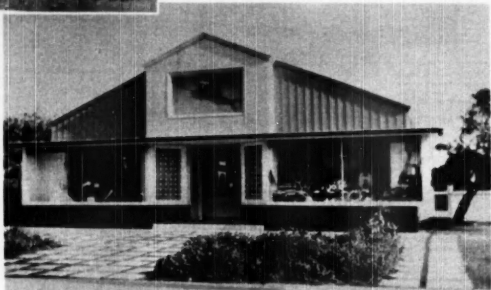
COMPLETE new front replaces the old. Contour of roof retained in the new design. Present masonry work painted and pointed
