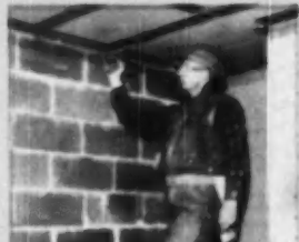
This worker is applying metal lath to a ceiling with a cigarette in one hand... thanks to his handy Bostitch T5 Tacker. Easy does it.
