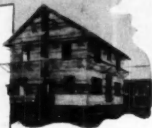
FASTENERS are nailed to studding at 14 inch intervals, preparatory to receiving panels
