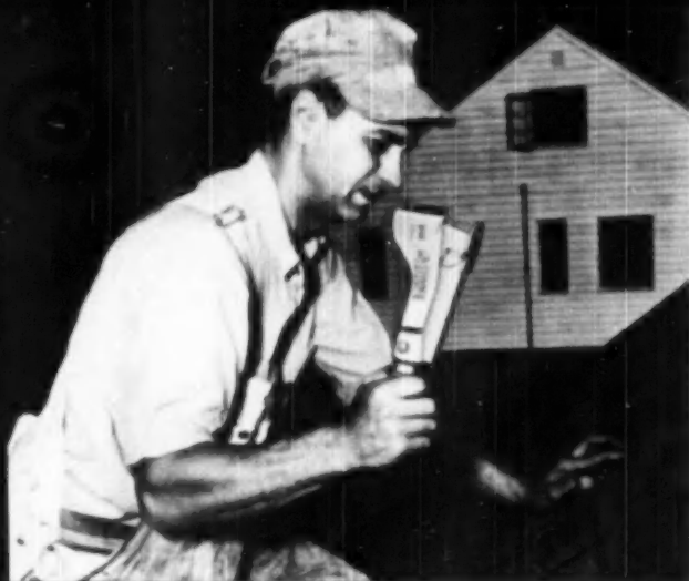
Applying insulation pads with Bostitch H2 Medium-Duty Stapling Hammer at top speed with much less worker fatigue than with hammer and nails.
