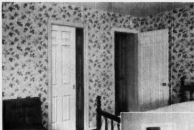
Bedroom closet door with Richards-Wilcox Vanishing Door Hardware. Note that the door does not interfere with the chair, and does not take up any passage space between the bed and wall.
