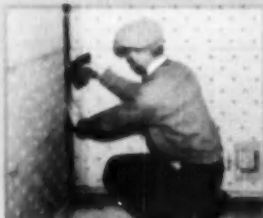
Self-fed staples speed work in corners where it would be slow and awkward to hold a tack or nail with the fingers.
