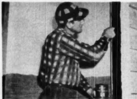
FIRST, brush heavy coat of asphalt emulsion on jamb and sill
