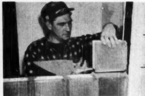
THIRD, lay the blocks in, position using full mortar joints
