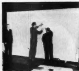
APPLYING 8x14-foot panel to studding by use of patented floating fasteners
