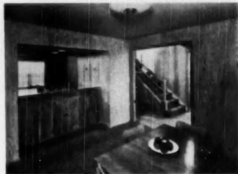
PRESIDENT Herbert Malarkey's office is now in oak parquet which gives wall surface an interesting pattern. Light color of oak plywood makes it one of the best woods for office paneling where light is a factor
