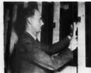
FASTENERS are nailed to studding at 14 inch intervals, preparatory to receiving panels
