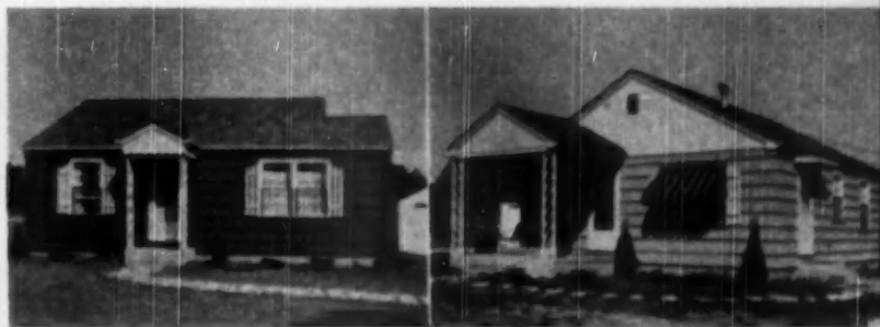
FLAME , left and right above, are for those homes built with fabricated sections, pre-cut lumber
