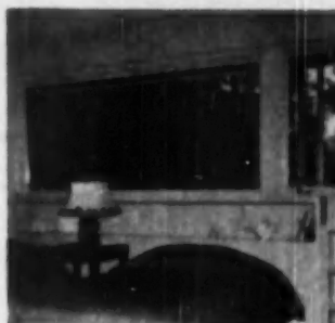
WALL extension under window sill in master bedroom provides shelf area above head of bed. Shelf occurs across entire wall
