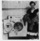
te dry six pourds of clothes in 15 to 25 minutes ready for ironing. For bane dry clothes, 30 to 35 minutes are required. Finish is white, high-luster baked enomel with red plastic trim and throme. Over all dimensions are. height-39 inches, width-31 inches, depth-27 ½ inches, Mamilton Manufacturing Company, Two Eivers, Wis.
