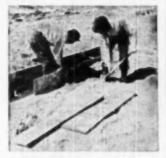
FIRERGLAS Stab Edge Insulation being placed around perimeter of Levilt house. 12x48-inch hourds are installed vertically
