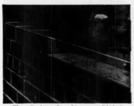
When morter is spotted on only one corner of the brick, slushing seldom fills the voids.
