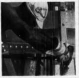
STUDS for siding material are installed before exection of corregated aluminum
