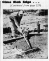
NEXT step is to smooth the concrete over insulation and radiant heating colis
