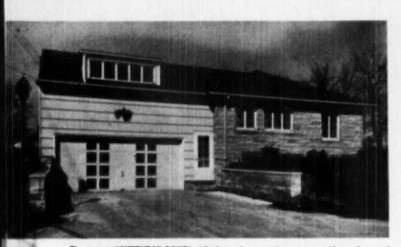
The two-car "OVERHEAD DOOR" of flush wood construction, gives a wide, unohstructed opening, fhe door is equipped with the model "H" electric operator with radio type control
