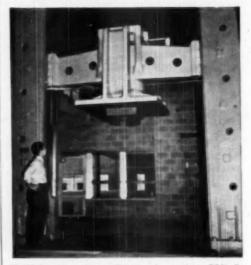
TESTING machine of one million pounds capacity at PCA's Research Conter crushes concrete specimens to determine strengths
