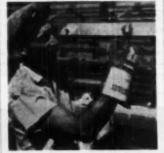
AFTER installation of stude, aluminumcolored asphaltic-base paint is applied around stude for long-term protection
