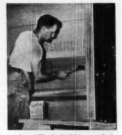
. . . but "Zinclad's" biggost help to the industry is offering a neil actually dipped in molten zinc, not just galvanized, for a coating that will outlast the building itself.
