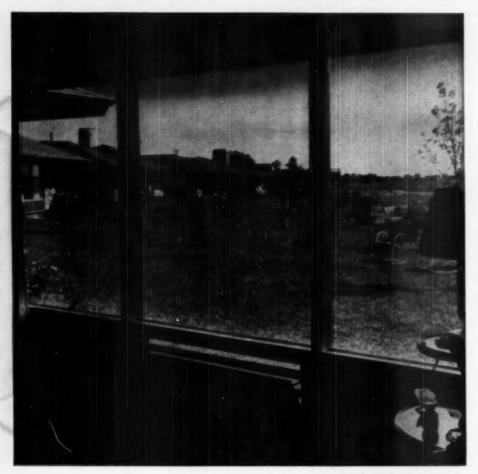
IN MANY RANCH-TYPE houses the trend is toward a fixed window wall, with houver-type ventilator. Here's something that homeowners will appreciate. For this construction, offered by Solar Air-Flo, Inc., Elkhart, Indiana, gives an unobstructed view through the Pittsburgh Twindow panels, with adequate ventilation and insulation. And louvered sections may be placed at top, bottom or sides of Twindow panels, according to design requirements.
