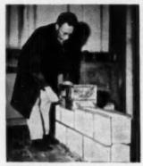
**INVENTOR** Jack J. Wegner demonstrates use of mortor spreader designed to reduce waste in laying concrete block up to 50%
