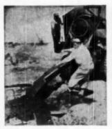
CONCRETE is poured over top and an top of two rows of the insulation to enclose it
