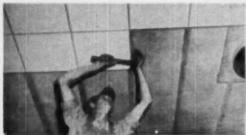
INSULATING board tile being applied to furring strips with concoaled nulling, it is especially important that framing or furring strips for tile conform to size of units used
