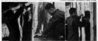
THIS TYPE of biunket insulation is compressed for uniquenest. When installed, it is cut to right length, stupied to the top plate and then stretched to ficer plate and suspise there with fiber strips both up and licition for firm attachment. It is then singled to sides of stude to provide air opens with the reflective foil on the interior, warm side
