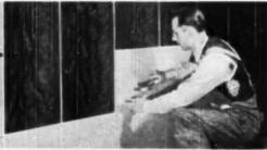
INSULATING board into its applied with the long edges at right angles to framing or furring. When small areas are to be filled out, insulating loth must be used; not wood
