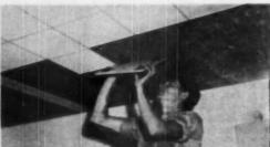
SOME manufacturers have worked out special clip systems and interlocking joints for installing insulating tile. In this photo the tile is being applied with a special adhesive
