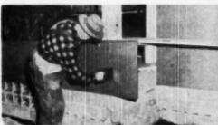
INSULATING board sheathing is applied by notifing to intermediate stude first with the notic about six inches opent. Notic around edges are spaced three inches apart
