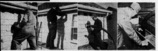
IN INSTALLING blow-in fill insulation in existing structures. access to appear between study is made by removing small sections of the exterior finish and then drilling holes in the sheathing. In every stud section a plumb bob is dropped inside to locate any
