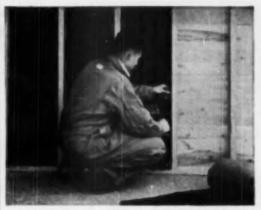
APPLYING INSULATION TWICE AS PAST is a relatively every matter with Bostish self-feeding stopling howners. One-blow, one-hand operation leaves other hand free for faster, better placing of material.
