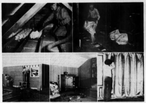
(6) LOOSE fill insulation being blown in: (7) Granular fill insulation being poured; (8) Insulating board sheathing; (9) Decorative insulating board on interior finish; (10) Reflective Insulation. Photos coursey; (6) United States Gypsum Co.; (7) Vermicullis Research institute; (3) and (6) Insulations Board institute; (3) The Statistication.
