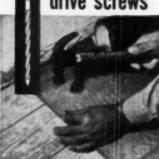
To make your linoleum underlays hold tightly and lay flat permanently, secure them with Hassall linoleum underlay drive screws. They are spiralthreaded and cement-coated for maximum holding power. Heads are flat countersunk type. Size: 11/4" x #3 ga. State quantity when writing for prices to:
