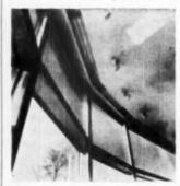
CLOSE-UP shows small slot opening around perimeter of false ceiling, from which warm air is forced downward to prevent forging of windows and to minimize heat loss
