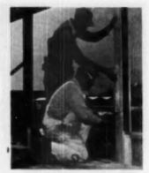
FACTORY-drilled mullion cover is held in place as a template while electric impacted drills 5/8-inch into the steel I-boam
