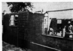
HORIZONTAL joints are accented in exterior wall of "Television House," These joints between concrete block are tooled
