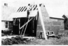
A "BOND-BILT" garage under construction. It is conventionally framed, with 2x4 stude, 16 inches O.C.
