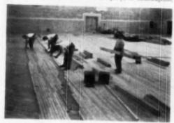
FLOORING, made by Connor Lumber and Land Co., is laid in record time in new Fond du Lac school. Called "Laytite." It is tongue and grooved on sides and ends. Here, no lengths under four foot were used in constructing the symnosium floor
