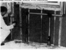
BATTS or blankets should always be worked carefully around sipes and conduits. Water pipes should be protected from treesing with insulation on the cold side but the vapor barrier retained on the warm side.
