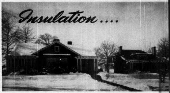
SNOW which disappears quickly from the roof of an uninsulated house is dramatic evidence of tramentous heat loss
