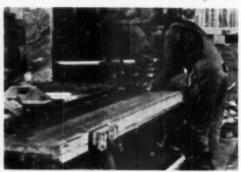
LOW platform of trailer permits use of power saw without climb ing. Natis and other supplies can be locked in trailer at night
