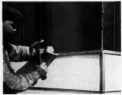
SHADOW lock system of installing shingles is used on Popular Home magazine house sponsored at Fair by United States Gypsum Co. Aluminum channeled strips, corner angles and hook natis are used to obtain deep shadow lines and distinct corners
