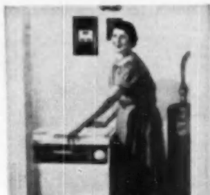
COMPACT Culligan Service Tank which provides filtered soft water is located in utility room of this home in Bonneyville Project, Pueblo, Colo., each unit of which has fittings for water softening service
