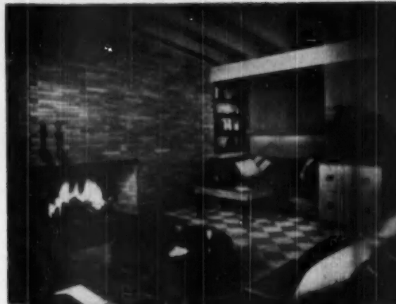
IN INTERIOR , masonry of both Roman ruffle brick walls is exposed. Fireplace, as shown in photo, is integral part of wall.
