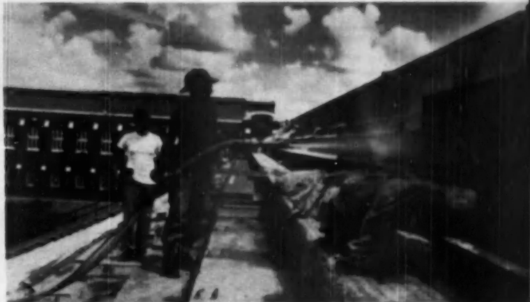
REPAIR of State College Stadium was simplified with pneumatically applied concrete
