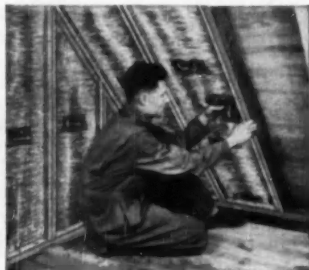
4 Flange stapled to sides of framing hold blanket permanently in position and also provide air space. Part of flange folds over face of framing to complete vapor seal.
