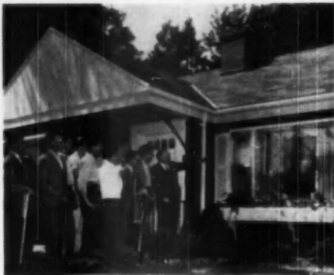
AT AN announced date and time the 12-foot fence was removed to reveal the completed house, fully equipped and furnished. The first week it was open more than 11,000 persons visited the highly publicized home
