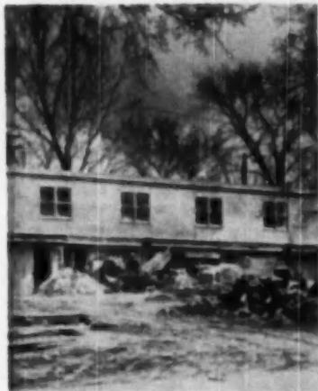
exterior finish of this wood-framed apartment
