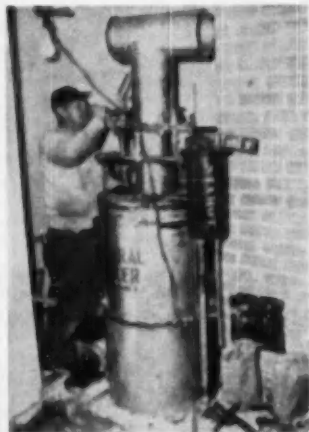
A WORKMAN completing assembly of the compact water boiler for the radiant heating system in Mystery House and others in the 70-house Green Acres project
