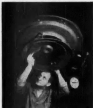
TRANE Louver Cone diffuser, suspended from unit heater, has spoke-like blades. Angle of blades can be set with fingers
