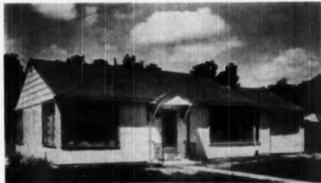
TYPICAL example of a home completed with Bldrok used for exterior walls. This home, in Fowlerville, Mich., is 28x54 feet, and was built at comparatively low cost
