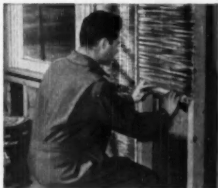
2 Snug fitting, many-layer KIMSUL blanket is then expanded to full length of stud space.
