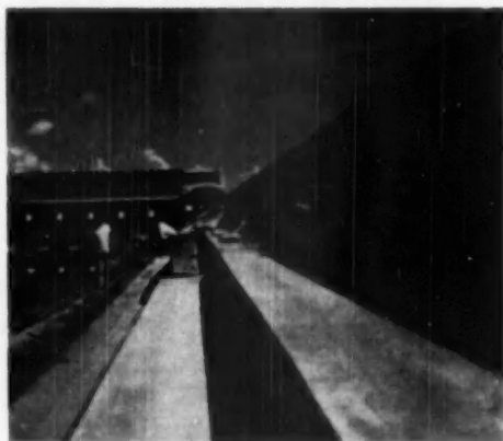
NEAT, smooth finish of the new surface of the floor adds not only to the appearance of college stadium, but to its durability as well
