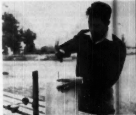
NAILS drive easily into the new panel
