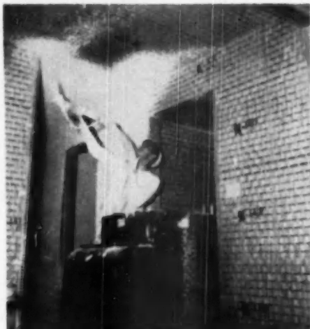
PLASTER made of light weight aggregates is sprayed on a paper-backed lath, K-Lath, by E-Z On Plastering Machine
