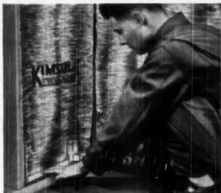
3 Staples through fiber strip attach end of KIMSUL blanket securely to floor plate. Stitched construction assures uniform coverage—prevents thick spots, heat-leaking thin spots.
