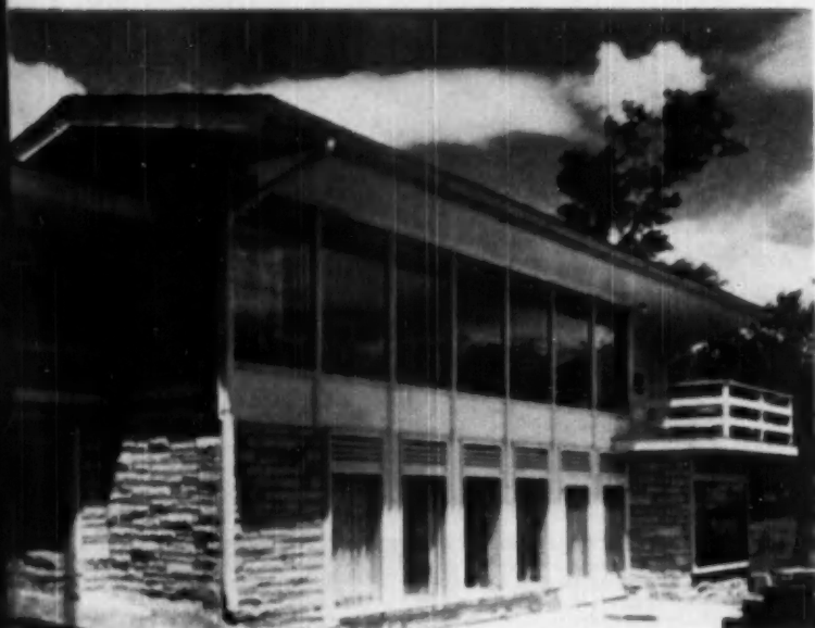
PARTIAL view of garden side of house, showing window walls to living and playroom. Ventilation of playroom area is controlled by horizontal louvers over window openings, with hinged panels on inside. Balcony overlooks swimming pool at rear.
