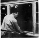
GLAZING stops should be applied carefully. Be especially particular to keep the acrows headed vertically and to leave the acrew head so the slot is vertical
