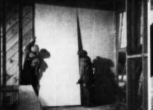
IN DOUBLE wullboard installations, first layer of panels is secured vertically
