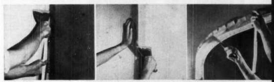
CORNER JOINTS are finished similarly to flat wall juints, as shown, left. Center, tupo is folded to cover angle, and is commended to estside carner. Outside angles of curved surface are toped as shown, right. Back of gypsum beard is scored to allow bead
