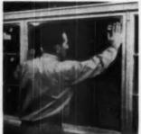
DOUBLE-glosed unit is put into place on the setting blocks and qually pushed into position aquinst compound covered steps. Steel frame gives the unit added strength making the hundling easier. With slow but firm pressure the steel framed unit is forced inward until all voids are filled
