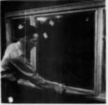
COMPOUND is applied to exterior glassing stops. Allow at least 16 lack of glassing compound between the steel channel frame and stop. An important factor to consider is that glazing compound and step should extend beyond edge of steel frame. This increases insulating qualities of the unit
