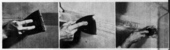
FIRST STEP in concealing wellboard joints is to apply cament to channel, as shown, init. Second, reinforcing tupe is imbedded in cament over insigh of joint, and third, right, encess cament is removed. Tupe then is covered with coment
