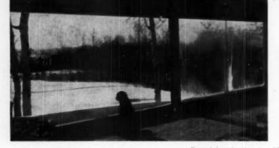
INSTALLATION of two types of glass in window wall' shown at left was made for the purpose of comparison during portial of entreme tomporatures. Large unobstructed glass area at left of picture shows an installation of hermetically-scaled double-glassed window. The opening at right is glassed with two lights of single
