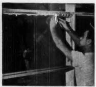
Window wall frame nailed into place, ready for insertion of either standard 451%"x251%" Thermospane units or aluminum projected type windows of like size.
