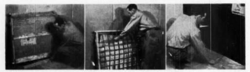
DOUBLE-glassed units are delivered to job its strong crates. First step is to till crate at slight angle, placing block in front. Remove one side of crate to start unpacking UNIT is protected on the inside by specially developed rigid cardboard web. The unit, with its stainless steel frame. in further protected by a heavy craft paper AFTER unit is removed from create, place on wedges and against wall. This permits steel frame to rest flat against wedges with weight of unit equally distributed
