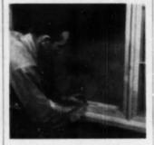
WOOD setting blocks 12-inch thick, one inch wide and about three inches long are placed in the position indicated by pencil mark on ince of inside stop. A 36-inch such width is used in this installation, thus the setting blocks are 9 inches to from onds
