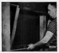
Aluminum ventilators of projected type are inserted into openings of wood frame in a hed of glazing compound. Wood screws hold them in place.
