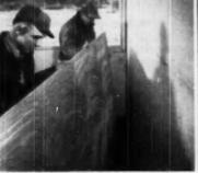
FACE LAYER in gypsum double wall system is "buttered" with a special coment
