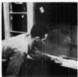
ADHESION of the gluzing compound helps to hold double-glazing unit in place. Howover. as a precoution, temporary stops should be placed on top and sides. Next stop in glazing is to fill in the wolds between the steel frame and the wood opening which is the 16 inch clearance allowed for setting
