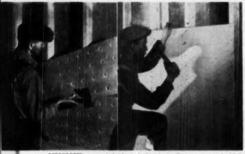
PERFORATED gypouns lath, identical otherwise in all respects to standard lath, as shown above, right, allows plaster to "rivet" to lath with mechanical key
