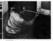
CHECK the window opening against the size of window unit. Unless specifically indicated on glass there is no top or bottom
