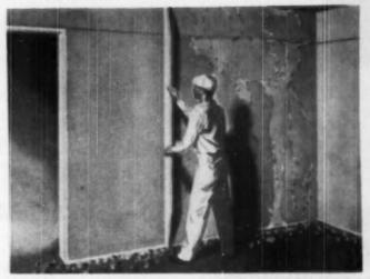
RODDING tool is used between grounds or screeds to develop proper thickness and plane
