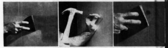
IN FOURTH stage a second cost of cement is applied over imbedded tape, and edges are feathered out, as shown, left. Center illustratics shows how natis are "dimpled." Before concealing natibends, make sure each board is tight against the framing
