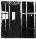
WALL FRAMING: 4x4 members at head and jambs. Bracing cuts into studs
