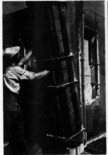
CORNER form developed by Pollman can be handled by one man, and adjusted to any angle from 30 to 90 degrees
