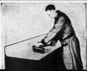
Contact pressure with an ordinary hand roller assures a perfect band. Note how VERSIBOND can be coved.
