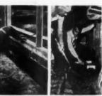
EDGE INSULATION in position at wall
