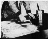
A uniform coating of cement is applied to the rubber backing of a VERSIBOND sheet likewise, the underlying surface is also
