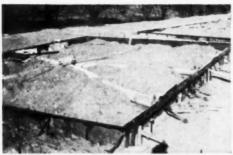
HEATING ducts, which are imbedded in concrete slab floor, are easily assembled by one man, Curved joints are of light metal
