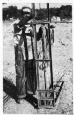
BENDING periect 90-degree angles in reinforcing rods is easy with this device made by Place and Company men. The rods are used at corners of concrete alab floors
