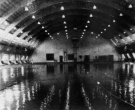
THE PROBLEM of constructing wide, clear spans with wood framing is effectively overcome by using glued laminated wood framing members
