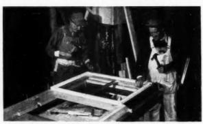
A HANDY jig in the Piace mill is used to frame aluminum windows. Framing members become the finished jamb in Place homes resulting in cost economies
