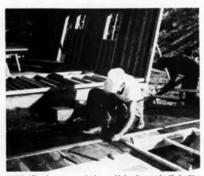
WALLS of Place homes are completely assembled on the ground, with sheathing and siding or shingles applied, then tilted upright into their proper positions
