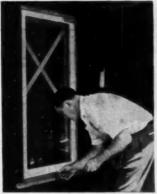
ANCHOR WINDOW — Pella Windows are completely assembled when they arrive. Just set the unit in the opening and anchor it firmly at the head and sill. Flange screw are furnished for this purpose.
