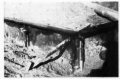
STREET curb forms are used for concrete slab forms. Hinged corners are securely held by an easily removed steel pin
