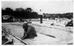
REINFORCING wire mesh is laid over the paper before the concrete is placed. Specialized crews handle all the concrete work
