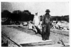
VAPOR resistant paper is placed over the leveled fill. Heavy rigid type insulation is placed around outer perimeter at slab
