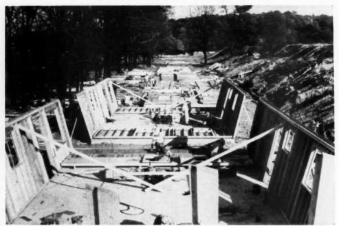
FROM concrete slab floor to finished framing is a fast step in Place and Company operations. Top soil is shown in pile, right
