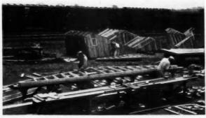
GABLE ends are completely assembled at the yards before they are hauled to the building site. All roof rafters are precut in shop and assembled at site
