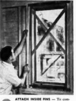
ATTACH INSIDE PINS — To complete the installation, apply the inside metal fins at head, sill and jambs. Fins fit under the lip of the stel frame and are nailed to the studding. This insures a tight weatherscal all the way around the window.
