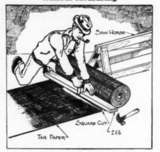
After tar paper, roll roofing, linoleum or paper are partially unrolled, a perfect cut can be made with little effort. Place the roll against a sawhorse or stepladder, and then take a straight 2x4 and hold it firmly against the roll as shown in the drawing. Take a sharp knife and cut along the edge of the 2x4. The cut will always be square.—Herbert E. Fey, New Braunfels, Texas.
