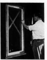
ATTACH OUTSIDE FINS — Next, attach metal fins at jambs. The grooved edge of the fin fits over the edge of the steel frame. The flat surface of the fin is nailed to the sheathing. Exterior trim can now be applied.
