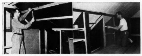
WHERE insulating board plank was applied to walls and celling 1 x 3-inch furring strips were natled to framing members AREA back of the knee wall was insulated and finished so it could be used for handy built-in storage shelves and cabinets
