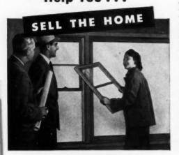
Show the woman prospect how R+O+W Windows can be REMOVED for washing or painting both sides indoors by pushing each sash to the left against spring pressure.
