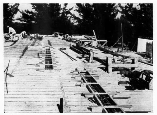
ROOF of Trails End Court. St. Petersburg, Fla., is made of Flexicore concrete slabs. Shown here is form for casting beams
