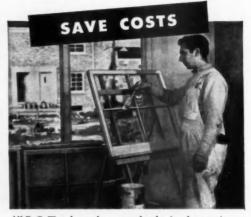
All R+O+W sash may be removed and painted at one time and in one location. Sash may be covered and stored away from frames to reduce breakage costs. Removable sash reduce reglazing and other maintenance expenses.
