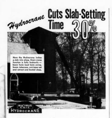
"With our Hydrocrane and four men we can place as many Flexicore slabs in eight hours as we used to in 12 hours with five men and an A-frame," says R. L. Hubler, Price Brothers Contractors, Dayton, Ohio. "During normal operation the crane sets a slab every minute and a half. Why, on one job we erected 7,000 sq. ft. of pre-cast in eight hours.
