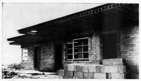
SLABS with prestressed steel reinforcement made 8-foot cantilevers possible. Finished ceiling is Flexicore, painted
