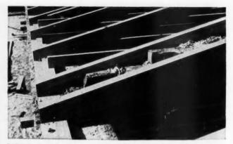
RAFTERS are nailed to wood plate (ordinarily a 2 x 6) bolted to top of the bond beam
