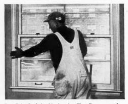
Free Paint Lock in this Amazing Way: Press exposed metal sash channels (at left) and sash in against spring pressure, paint lock is broken. A whole house takes just a few seconds.
