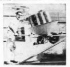
"Pow-R-Barrow" self-powered wheelbarrow will pull a full load up a 40 per cent grade. Compression acts as a brake on the downgrade. Speed on the level is a comfortable walking pace. Main advantage of the new machine is to eliminate most of the effort, rather than to materially speed up the operation. Air-cooled engine is mounted beneath bed and drives by firction on the tire tread, with simple controls all on the right handle. S and S Vending Machine Co... Dest, AB, San Jose, Colif.
