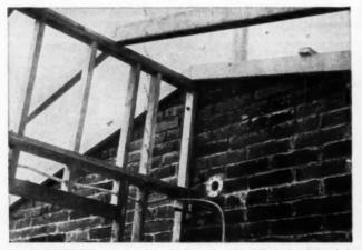
FRAME PARTITIONS are bolted to block walls with 18-inch foundation bolts APRIL 1951
