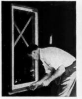
ANCHOR WINDOW — Pella Windows are completely assembled when they arrive. Just set the unit in the opening and anchor it firmly at the head and sill. Flange screws are furnished for this purpose.
