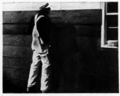
Leaving a two-inch overlap, a carpenter prepares to nail a panel of Masonite  $1/4^{\prime\prime}$  Tempered Presdwood over the insulation sheathing on the William A. Schraegle home at Parma, O.
