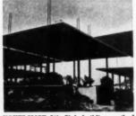
YOUTZ-SLICE Lift Slab building method was successfully used in first commercial test in erection of Trinity University administration building shown during construction
