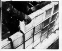
Installation speed goes up! The new gold stripe makes it easier and faster to identify inside top of block.
