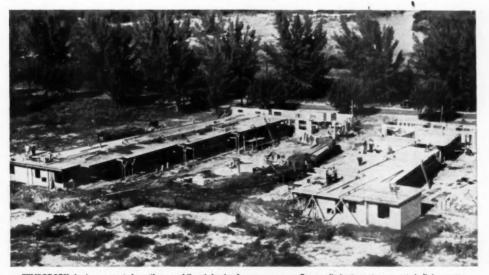
TEMPORARY shoring supported cantilevers while reinforcing beams were cast. Beams eliminate center supports in living rooms.
