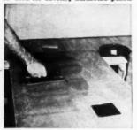
ADHESIVE is applied to hardboard panel with a saw tooth trowel
