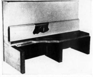
CUTAWAY MODEL of installation of metal wall base and stack supplying heat to base
