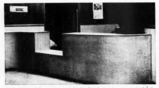
METAL MOLDINGS cover joints of this hardboard receiving counter in laundry AMERICAN BUILDER
