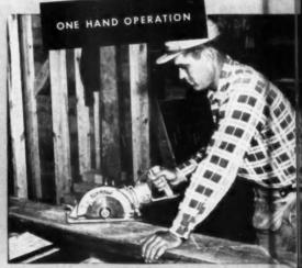
One-hand operation. "One hand on the saw, one hand on the work, and your eye on the blade makes accurate sawing easy with a SKIL Saw," says William Skaggs. That plan of action is demonstrated as he cuts a stair stringer with SKIL Saw Model 77.
