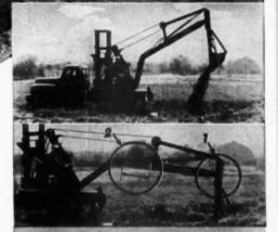
The Hydrohae is the only drogshowed with two appears ond distinct digging actions. The first is through a hydroxile rem lected between been and dipper handle. The second digging action comes from toisecoping the bases. This sectoalve toisecope feature eliminates maving drogshow! Back and forth when digging out boulders and accessing acress pipe and cable . . . permits digging a level, scellap-free track, meather reducing hand trimming.
