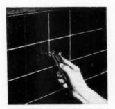
SCOREMARKS of tileboard are finished in a second color with a striping tool
