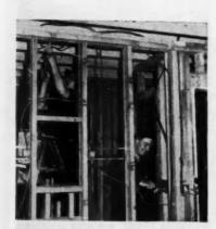
LIGHT-CONDITIONING begins while house is still in blueprint stage. Here crew is roughing-in wiring
