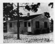
REAR VIEW of plan No. 1 (top of page) shows use of asbestos siding shingles
