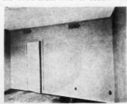
WATER FILLED this room in the Jayhawk Junior motel almost to the top of the door. The gypsum plastered wall has been washed down and is being allowed to dry. Trim suffered little damage, but hardware was removed from the door for repair
