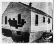
FLOOD CURRENTS TORE through and around homes at a rate of 35 miles an hour in some areas. Here, rapid currents washed the foundation from under this home and ripped some of the shingles from the structure
