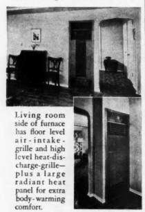
Back of unit also has cold-air-intake and warm-air-discharge grilles that provide circulated, uniform wholehouse heating.
