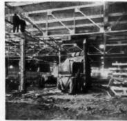
LARGE TYPE of temporary heating unit mounted on skids and designed for use in large open areas during construction of industrial structures in subfreezing weather
