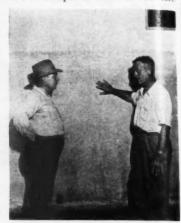
LLOYD H. YEAGER, general manager of the Gypsum Association (right) examines plastered wall in the Jayhawk Jur'or motel with Harry Lose, hotel official. Flood water level is apparent above the heads of Lose and Yeager. While water and mud stained the plaster, it failed to damage the wall otherwise
