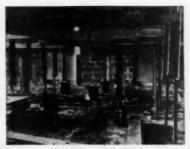
TEMPORARY HEATING units were used to keep this basement warm and also to heat floor above
