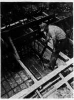
A pneumatic concrete vibrator designed to compact freshly poured concrete and to direct its movement as it is poured into the form, is called the Thor No. 521 Vibrator and is made by Independent Pneumatic Too' Co., Dept. AB., Sales Promotion Div., 175 N. State St., Aurora, III. Unit consists of 2½-inch d'ameter steel cylinder, 17½ inches long at the end of a five foot combination air and exhaust hose. Rotary air motor and vibrator unit are sealed in the steel cylinder.
