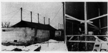
TENTS enclosing buildings under construction are hung on utility poles with ropes and pulleys which permit workmen to keep raising tent as the masonry work brings walls higher
