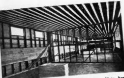
Interior view of school under construction. Note how wood collateral is nailed directly to metal framing.
