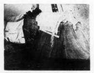
TARPAULINS or other suitable coverings are used in extreme weather to protect workmen and green masonry work
