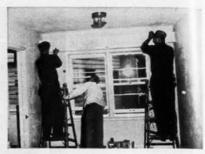
COMMERCIALLY AVAILABLE valance unit, one of seven manufacturers' equipment now available to builders, requires only mounting. The shielding board on the valance in the Dubuque Light Conditioned home slips easily into place, as shown above
