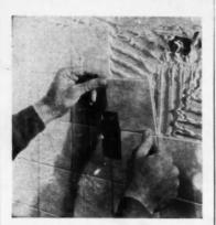
HOW the tile is fitted around sockets
