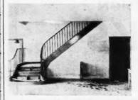
FLOOD DAMAGE is apparent in this picture, but the plaster suffered no permanent harm. Redecoration, however, will not be attempted until the plaster is reasonably dry. Care will be exercised, too, that the structure is dry throughout before repairs are undertaken
