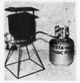
Designed for winter building is the new "Partable Heater". It delivers 40,000 B.T.U.'s and is capable of raising room temperatures 50 degrees in 20 minutes. The lightweight, 55 pound unit is easy to carry and its operational cost is estimated by the manufacturer to be \$1.00 a day. The heater is sold on a money-back guarantee, with a 30 day trial period. Manufactured by The Portable Heater Co., Dept. AB., Box 444, Painesville, Ohio.
