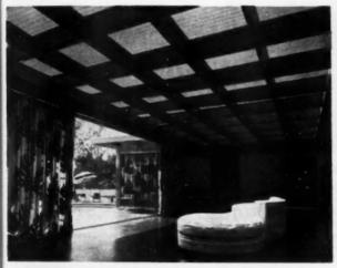
WHOLE ROOFS of Alsynite need only the lightest supports. Ideal for sun porches, greenhouses, barbecue shelters, etc. Alsynite weighs only 8 oz. per sq. ft.
