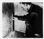
FIRST step is to measure for leveling point and to square and plumb all corners
