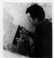
MASTIC is applied to the wall first in a vertical and then in diagonal pattern
