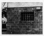
TWO gloss block designs were used here in combination, the clear block allowing vision with no loss of insulating quality
