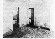
GYPSUM WALLBOARD performed well in the flood area. Stained and bruised in a few places, the wallboard in this home will be as good as ever after it is washed down and allowed to dry. A few minor repairs will be necessary. Mud left by the flood waters covers the floor of the home
