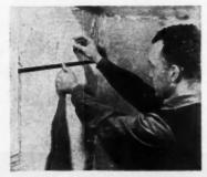
WHEN all of the tile is interlocked in position, feature strip is then applied
