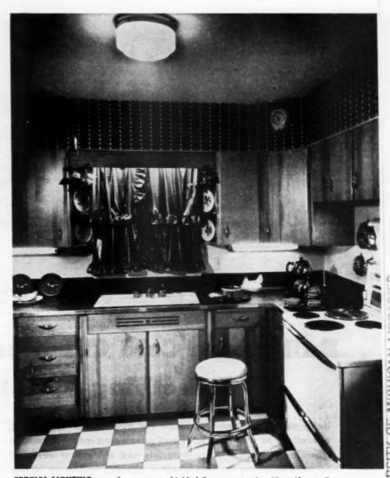
SPECIAL LIGHTING over the range, a shielded fluorescent unit with a 40-watt fluorescent tube, is mounted 58 inches above the floor to assure generous lighting over the entire range top. Lights over work counters (one 20-watt fluorescent tube for each 25 to 30-inch length of work counter) are attached to the bottom edge of upper cabinets
