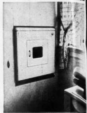
Automatic washer in the basement of home of Bernhard Dahl and Son West Coast builders (see page 158, September American Builder) is elevated two feet from floor for greater convenience. Machine is anchored to a heavy supporting timber frame-work concealed by the panel placed below the unit.
