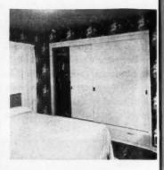
View in master bedroom showing the installation of a double acting sliding closet door unit. Note that doors can be reversed in position with ease. Drawers below provide a handy place for storage
