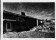
Partial view of rear elevation. Higher level at porch conforms to the street front. Rock garden planting covers the terrace between the two levels. Canopy over basement door is at floor level. Joists are extended to form the supporting members. Above grade windows supply ample light to basement area
