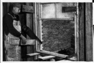
Square the frame and shim at these 7 places. Saw off shims flush with frame.
