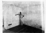
WASHED DOWN after the flood waters receded, these gypsum plaster walls in the Nod-Away motel on Highway 24 in Topeka, seems as good as new. Water line in this room was about level with this 6-foot tall man. Flooring suffered some damage
